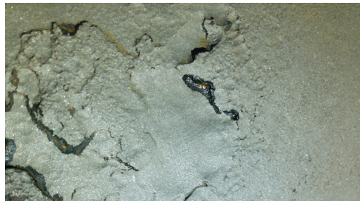
Severe corrosion and pitting was discovered when tape was removed, and the pipe was sand blasted.
