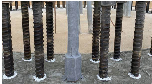
Trial application of the Denso ColorTape which showed how easily the tape conforms over irregular shapes.
