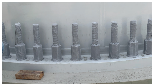
Recently installed Denso ColorTape on 76 exterior anchor bolts for tower.
