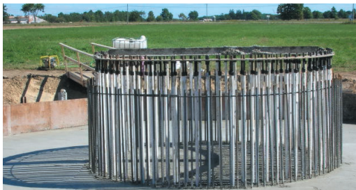
Rebar rods being installed on site.
