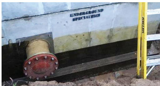
Denso Hi-Tack Paste and Tape is applied from the bottom up.
