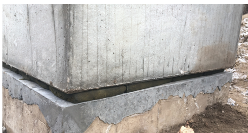
Densyl Mastic is laid upon the prepared surface in preparation for the box chamber.
