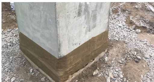
Hi-Tack Tape is applied 6" below to 6" above the joint and will provide a permanent flexible water-tight seal.
