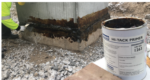
With the chamber in place, Hi-Tack Primer is applied in thin uniform coating.
