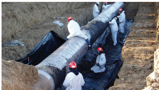
Removal of old coal tar enamel coating.
