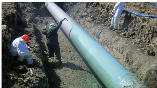
Pipe being spray applied with Protal™ 7200.
