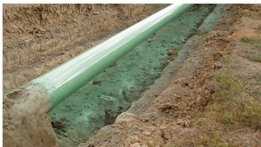
Section of pipe with newly coated Protal™ 7200.
