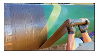
6.6 Ensure the wrap is completely saturated and then immediately begin wrapping compression film over the Denso Bore-Wrap quickly and with tension applied.
