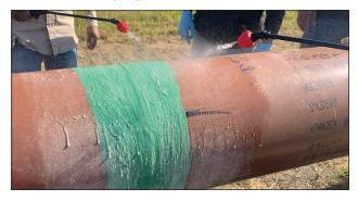
6.3 Denso Bore-Wrap is a water activated wrap. It is necessary that water is continuously sprayed onto the surface and underbelly of the roll as it is being applied. You cannot oversaturate the material, however insufficient water will slow the reaction and reduce product performance.
