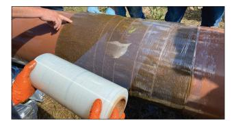
6.7 Once fully compressed, use the perforating tool to puncture the compression film. This will allow for excess resin, moisture, and CO<sub>2</sub> from the reaction to escape. Perforate using enough pressure to get through the compression film but not through the layers of Denso Bore-Wrap.
