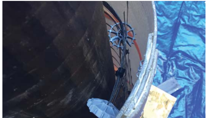
The SeaShield C-Grid® 450 with spacers that provides strength to timber piles prior to the SeaShield grout being poured.
