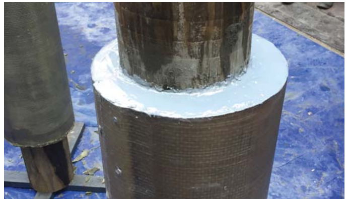
Completed SeaShield Series 400 System with freshly poured SeaShield 510 UW Grout protecting and strengthening a timber pile.
