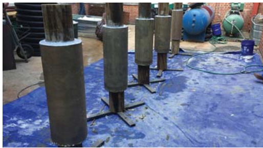
Repaired timber piles with the SeaShield Series 400 system.
