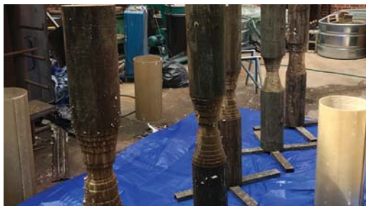
Hourglass shaped timber piles prior to installation of repair system.
