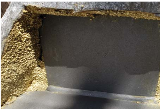
The surface of the structural steel column base immediately after removing the system that was in service for 12 months.
