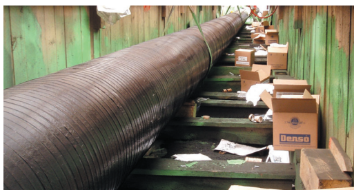
30" gas line protected with Protal™ 7250 overwrapped with Densopol™ Tape
