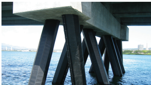
Series 2000HD protecting octagonal piles.
