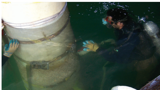
Pumping 550 Epoxy Grout.
