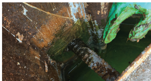
Denso Hi-Tack Paste is first applied to the tie rod to displace moisture and prevent rusting.
