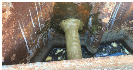
A tie rod fully protected with the Denso Petrolatum Tape System to prevent rusting.
