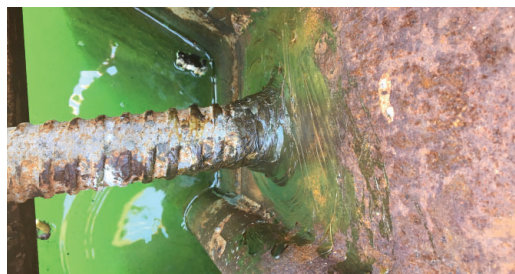
Densyl Mastic is used to seal the cavities to prevent water infiltration.
