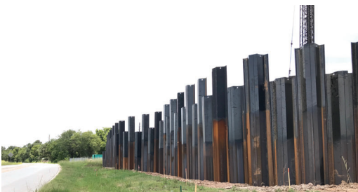
Sheet Piles coated with Protal™ 600 CTE being driven into place.
