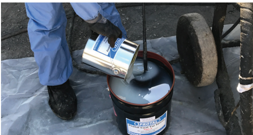
Protal™ 600 CTE Part “A” & “B” being mixed prior to the spray application.
