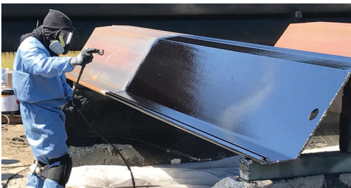
Application of Protal™ 600 CTE using a single leg airless spray pump.
