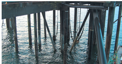
The wharf is supported by 20 year old steel pilings.
