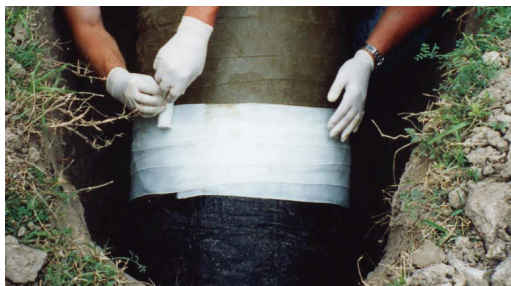
Denso Glass Outerwrap applied spirally over the Densyl Tape.
