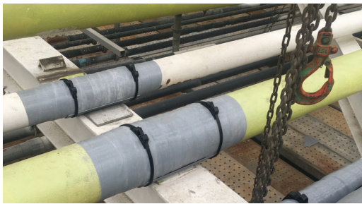
Denso ColorTape, Denso Glass Outerwrap UV, and FRP Spacer held in place by strapping.
