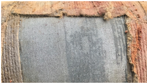
After 1 year, a field trial splashzone test with petrolatum tape & Glass Outerwrap reveals steel surface in perfect condition with no corrosion.
