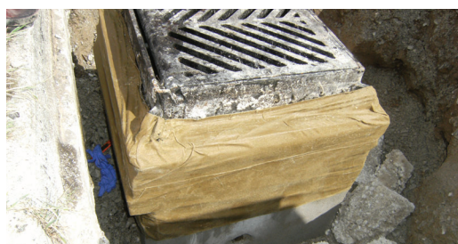
Structure, risers and frame of a catch basin quickly wrapped to prevent erosion corrosion.
