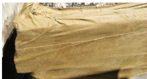
Denso Petrolatum Tape is loaded with material so will remain water proof even when concrete below cracks.
