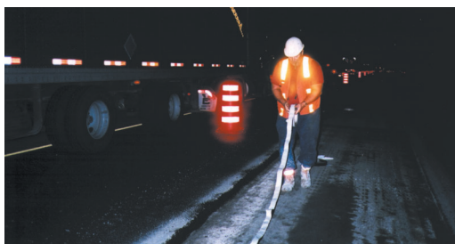
Densoband™ comes in several sizes. 15mm x 45mm x 6.5m rolls were used on this project.
