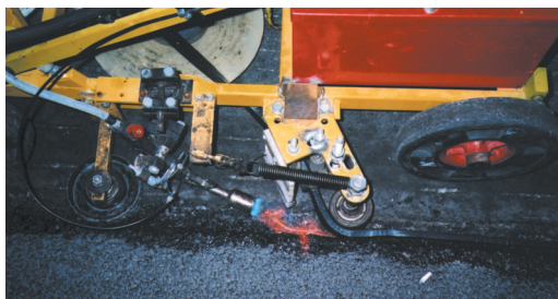
Applying Densoband™ at 360metres/hour with the special Densoband applicator machine.
