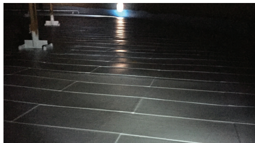
Pipeline storage company, 220' fuel oil tank, outside Albany, New York, on the Hudson River.
