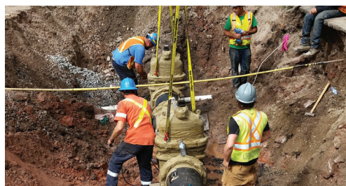
New water valves being protected by Denso LT Tape.
