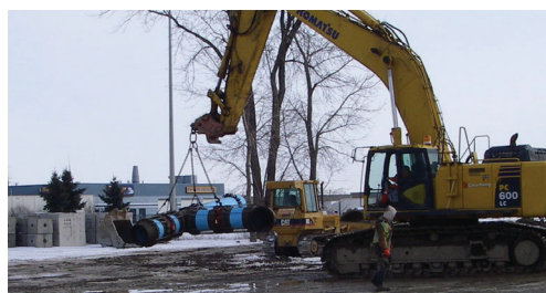
Water pipelines, with Denso LT Tape, being transferred.
