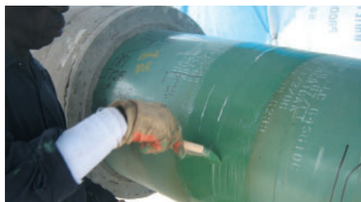
Protal™ 7200 brush applied to 30 mils at 180°F.
