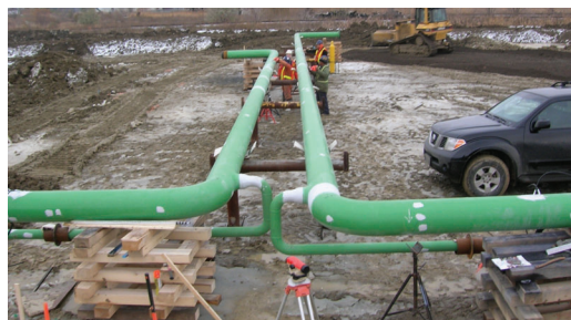
Holidays FBE pipe repaired with Protal 7125.
