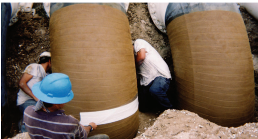
Denstyl Tape and Denso Glass Outerwrap is easily applied by hand and requires no special training or equipment.
