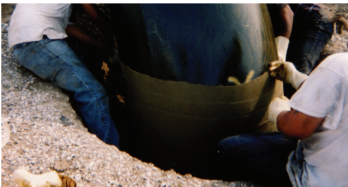
Denstyl Tapes provides long term corrosion protection to pipes, flanges, valves and related surfaces.
