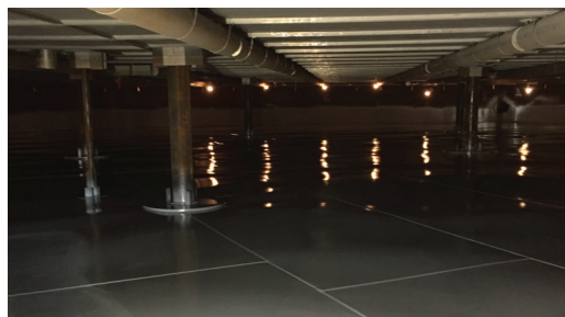
Fully cured Archco™ 476 is an excellent coating for crude, gasoline and other pipeline commodities.
