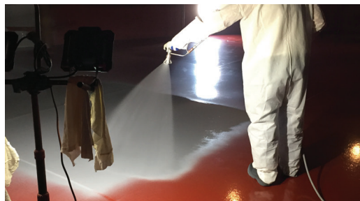
Archco™ 476 being sprayed applied over Archco™ 400.
