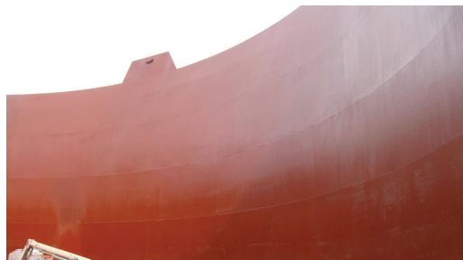
Open top tank, side walls primed with 400.
