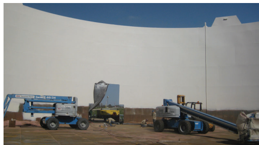
Open top tank, side was coated with 400 and 450 gray.
