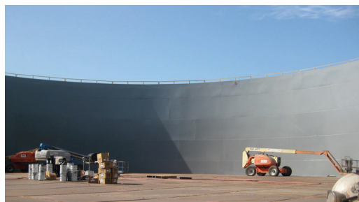
Open top tank, side was coated with 400 and 450 gray.
