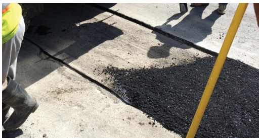
Application of the new asphalt road surface.
