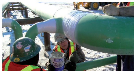
Application of Protal™ 7125, low temperature pipeline coating.
