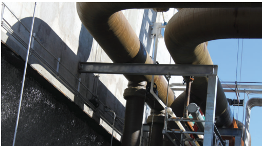
Denso Paste S105 and Densyl Tape applied to all straight pipe and bends.
