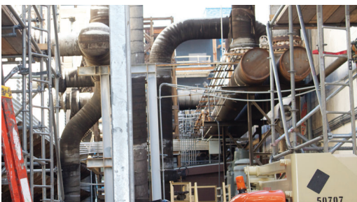
Denso Petrolatum Tape System applied 30 years ago to the old cooling tower and still performing well.
