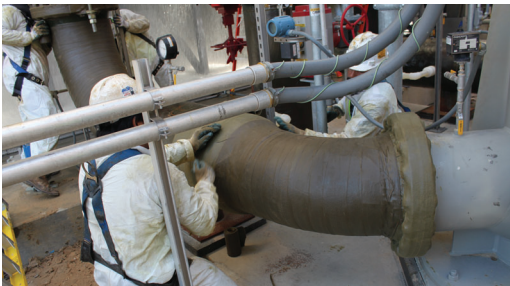
Denso Paste S105, Profiling Mastic and Densyl Tape applied to all flanges and valves.
