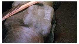
Completed application of one many valves and meters with Denso Petrolatum Tape System.
