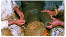
Densyl Tape is applied over the smooth contours of the Denso Profiling Mastic.
