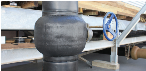
Weathershield 15 brushed applied onto Densyl Tape protecting a valve flanged as a top coat.
