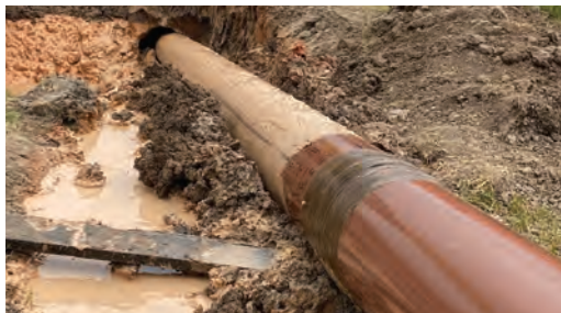
The first weld joint after exiting the bore hole.
