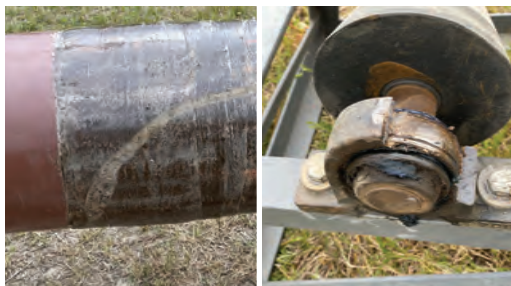
Denso Bore-Wrap® protecting the underlying coating after bearing failure.
