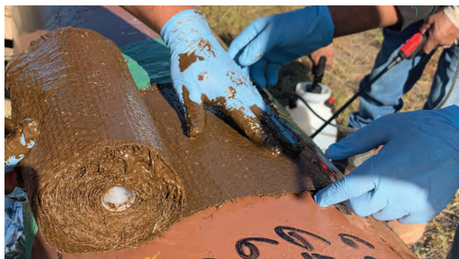
Denso Bore-Wrap® being applied over Denso Protal 7200™.
