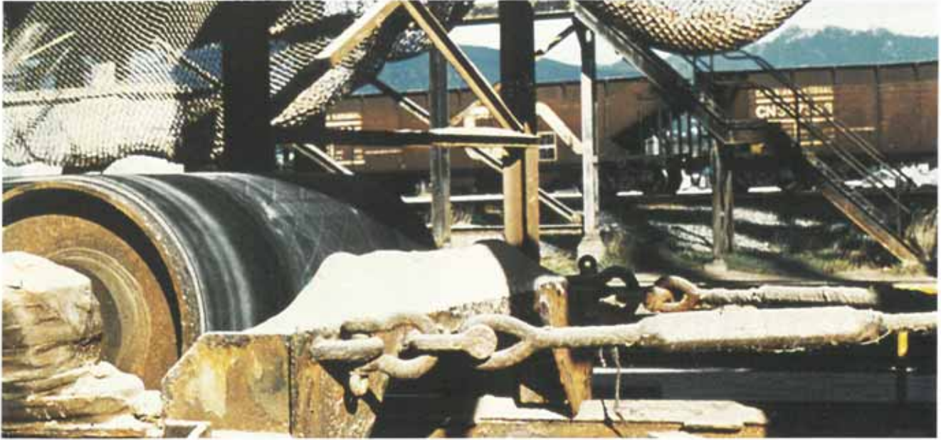
Denso wrapping protects from chemical corrosion such as potash . . .
