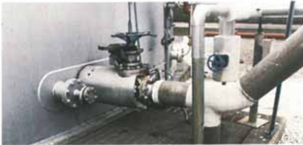
Tank outfall pipe in below grade sump ...
