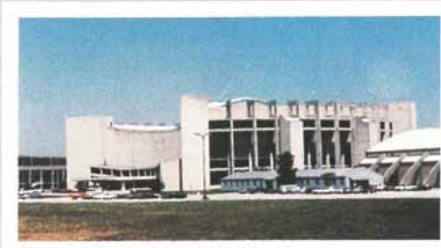
The Assembly Hall.
