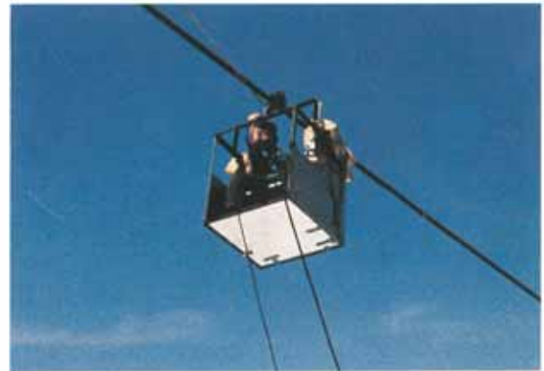
Up aloft applying Denso Tape.
