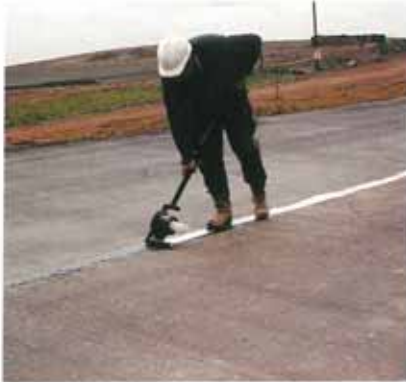
Tok Paving Tape applied after priming.
