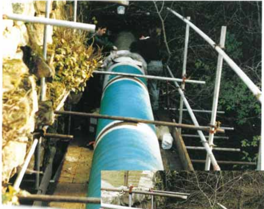
Covercoat coating in progress.
