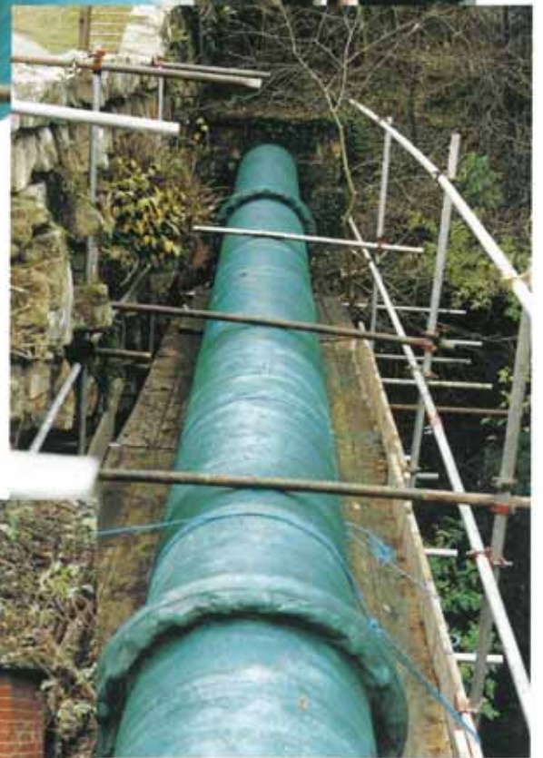
Completed Covercoat protection.
