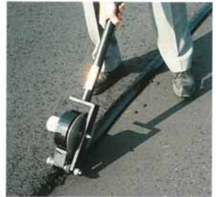
Tok Edge Sealing Tape applied with Tok Tape Roller.
