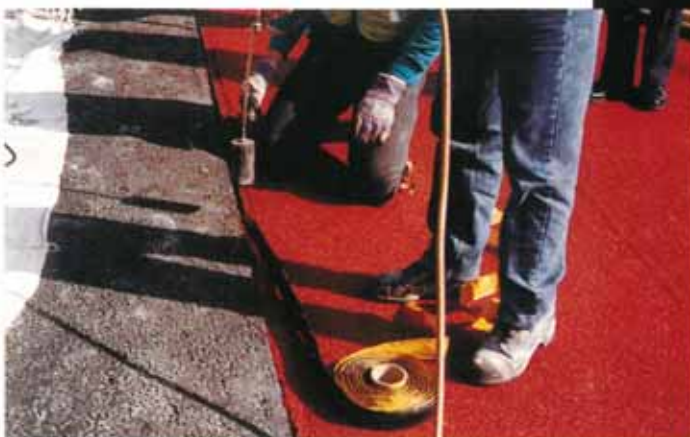
Tokband Spezial applied to the vertical joint face.
