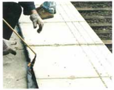
Tokband Spezial is applied to platform kerb edge.
