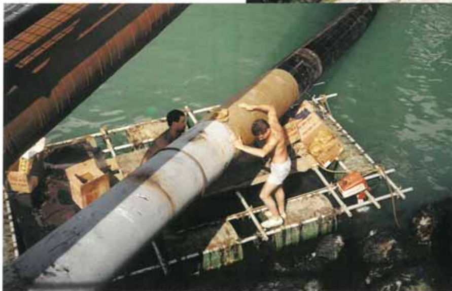
Initial Denso Marine Piling Tape wrap.
