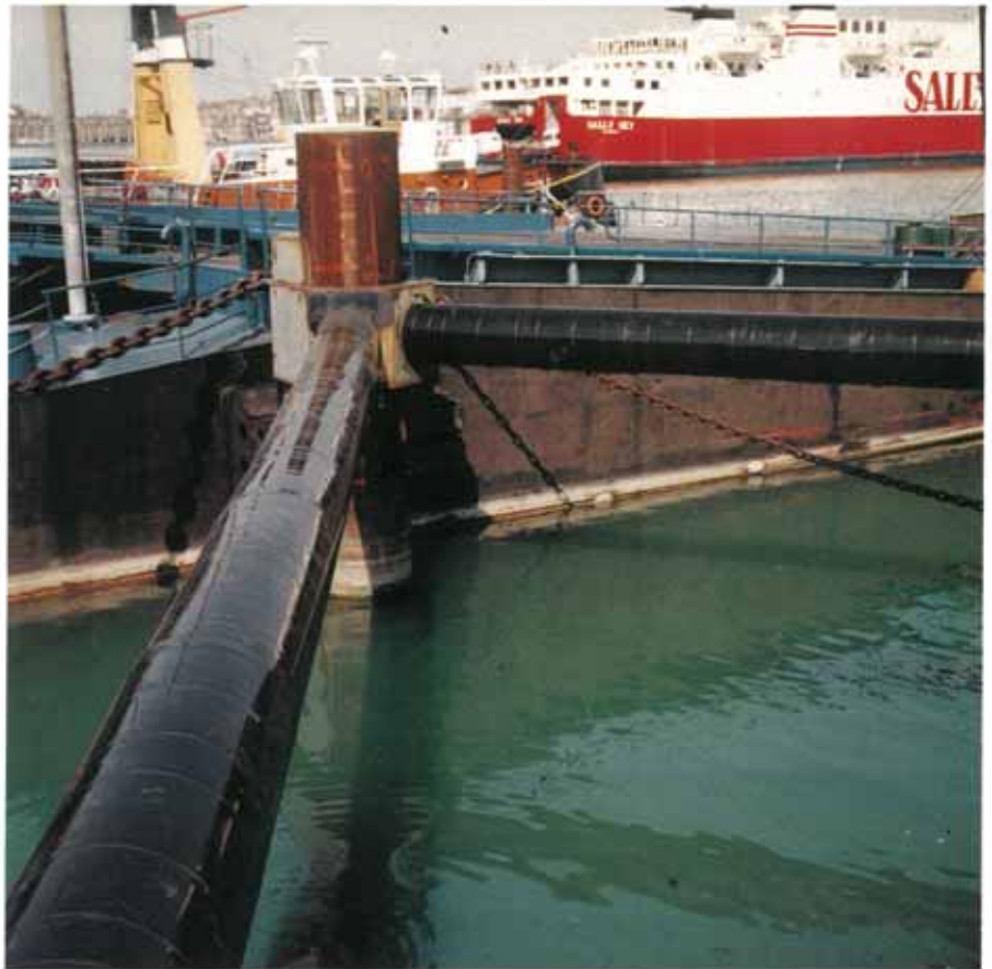
Upper Horizontal bracings finally protected with black polypropylene SeaShield covers.
