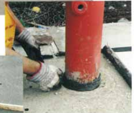
Tokstrip was also applied to metal lump bases prior to asphaltting.
