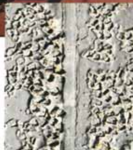
A flexible waterproof joint.
