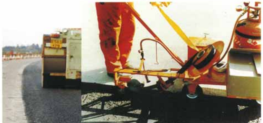
Tokband Spezial applied to vertical joint face with 'Tokker' machine.
