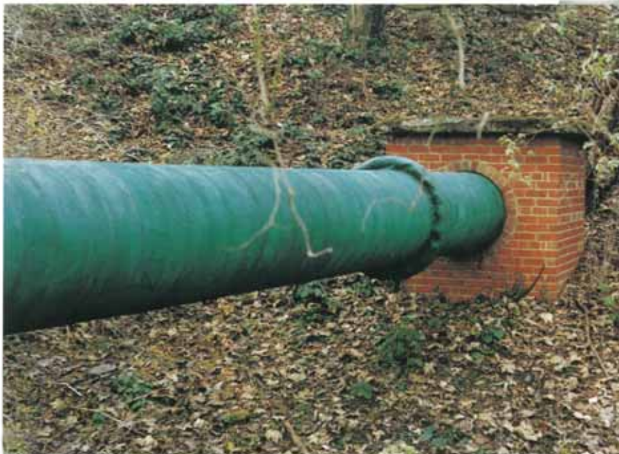
Completed Covercoat protection.
