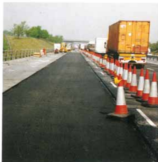
Tokband Spezial in place prior to asphaltting.
