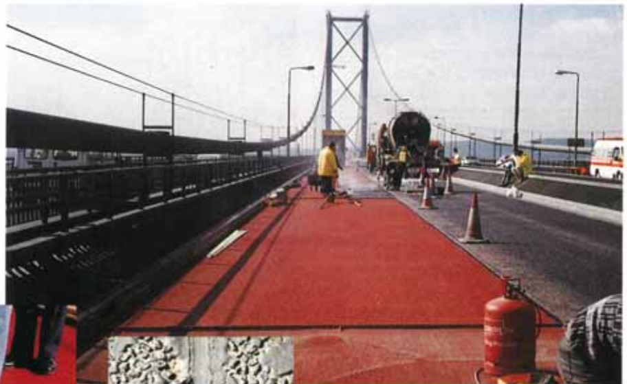
Asphalting in progress.
