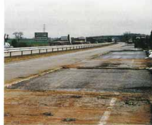
Damaged bays removed and base courses in place.
