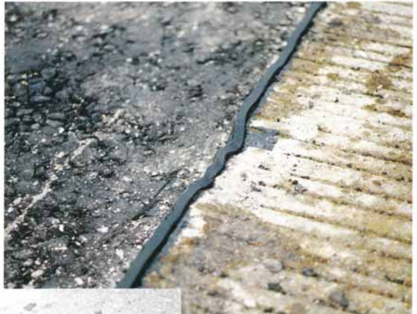
Tokband Spezial in position on the vertical joint face.
