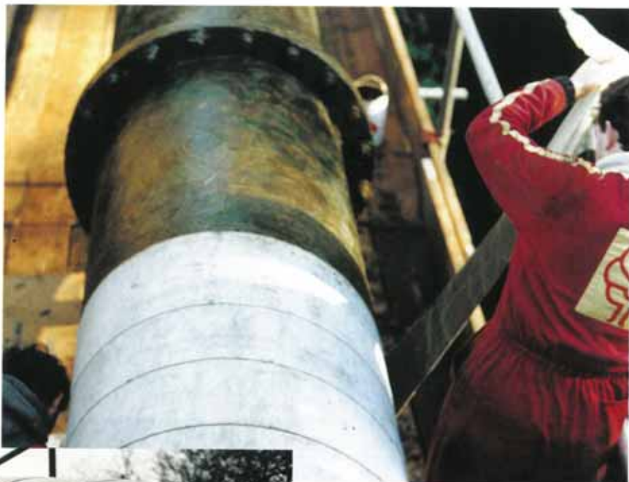
Application of Denso Covercoat Tape.
