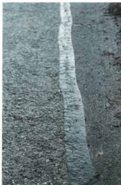
Tape in position.
