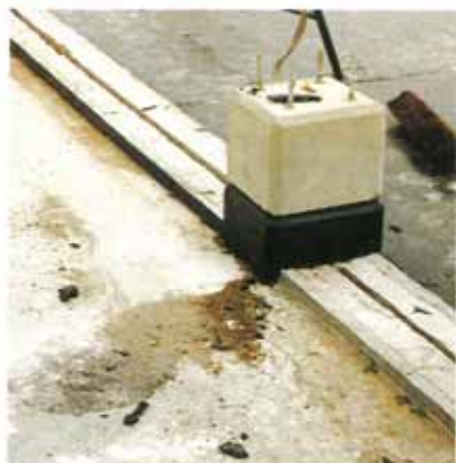
Tokband Spezial applied to concrete drainage channel.
