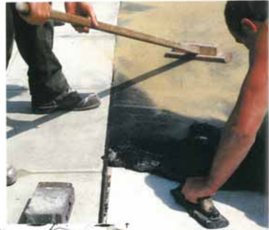
Tokband Spezial is applied to platform kerb edge.
