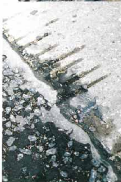
The finished joint.
