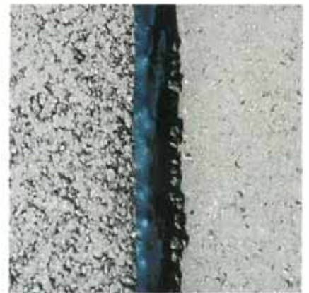
Close up of tape in position prior to asphaltting.
