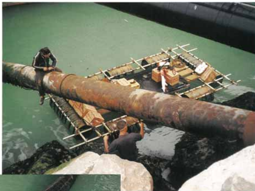
Raked bracing undergoing cleaning.
