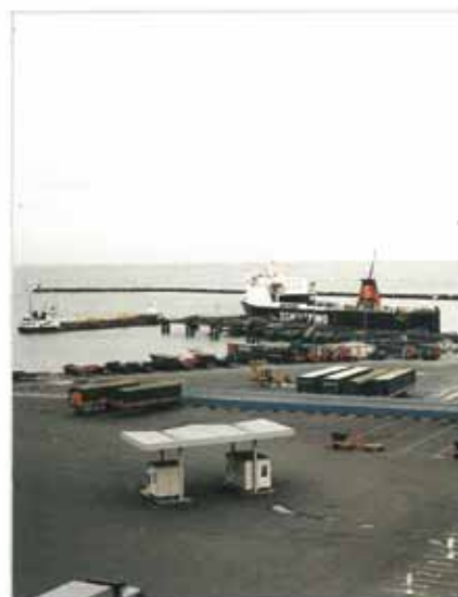
Port Ramsgate Ro-Ro terminal.
