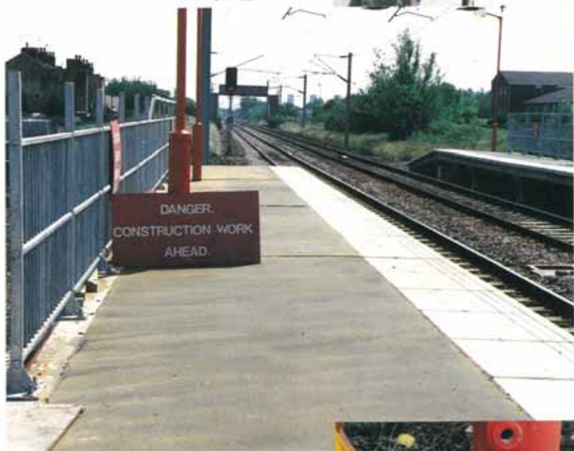
The finished platform.
