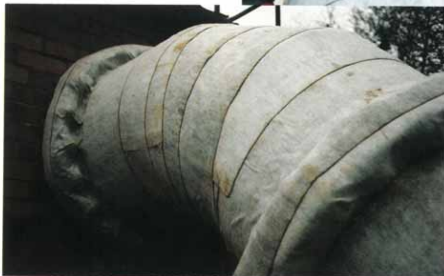
Tape copes easily with bends and flanges.
