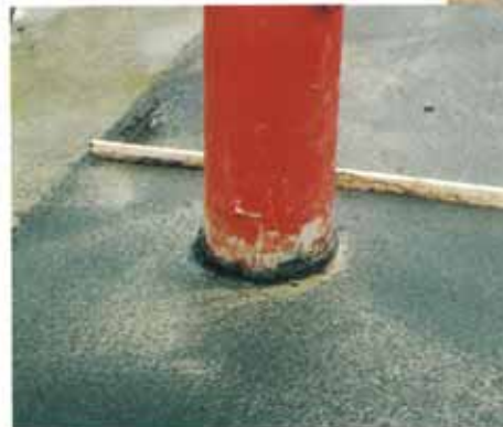
Tokstrip was also applied to metal lump bases prior to asphaltting.
