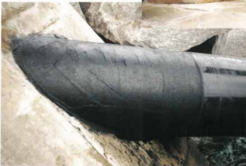
Finished protection consisted of two coats of solventless epoxy compound.
