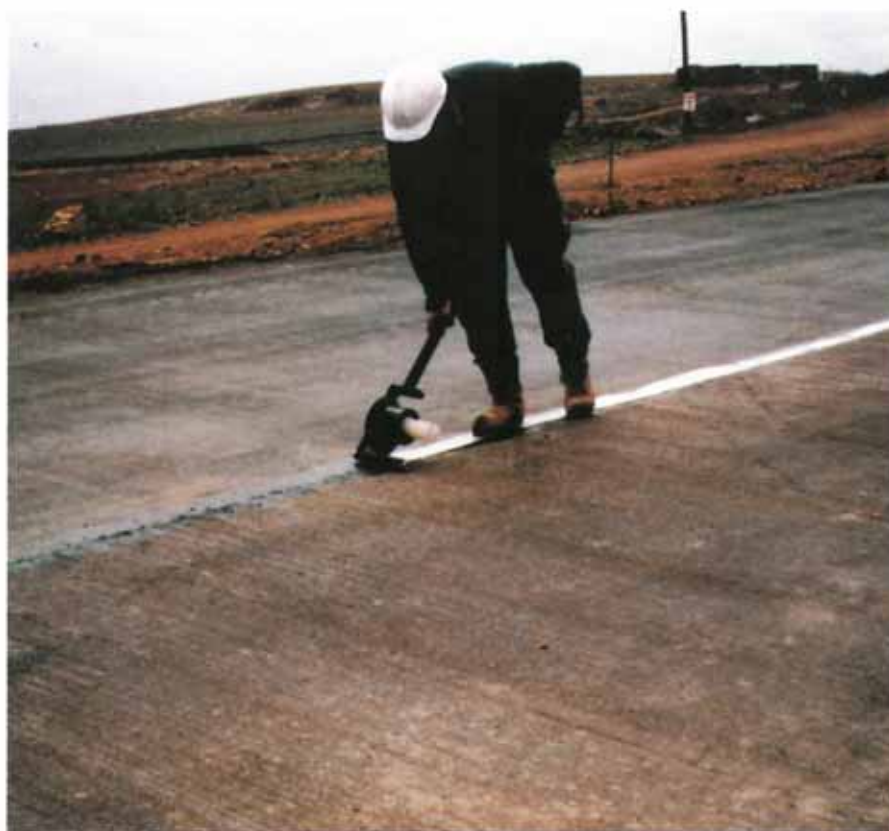
Application of Tok Paving Tape using special applicator machine
