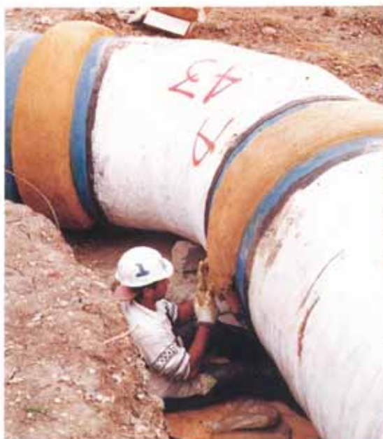
Easy to apply Denso Profiling Mastic.
