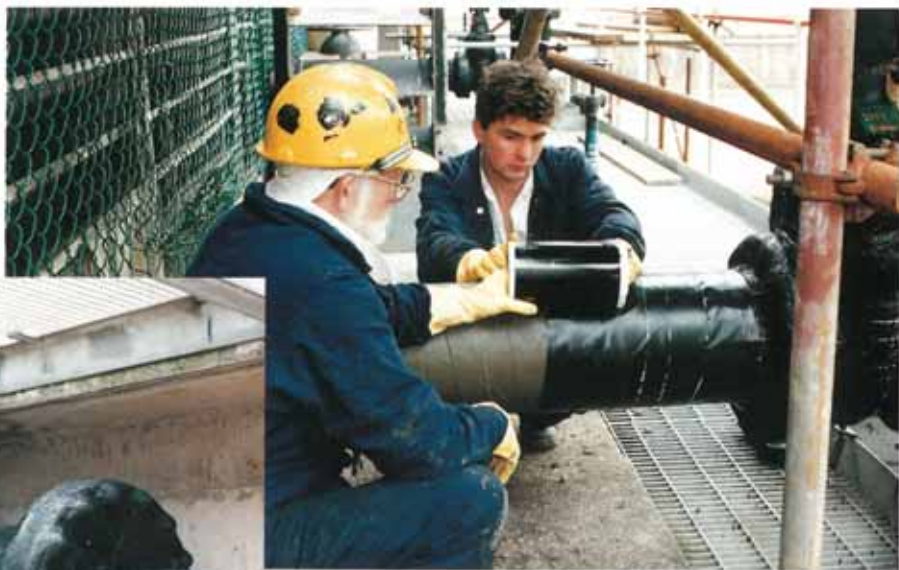
Above: Denso Tape overwrapped with Densoclad 40.
