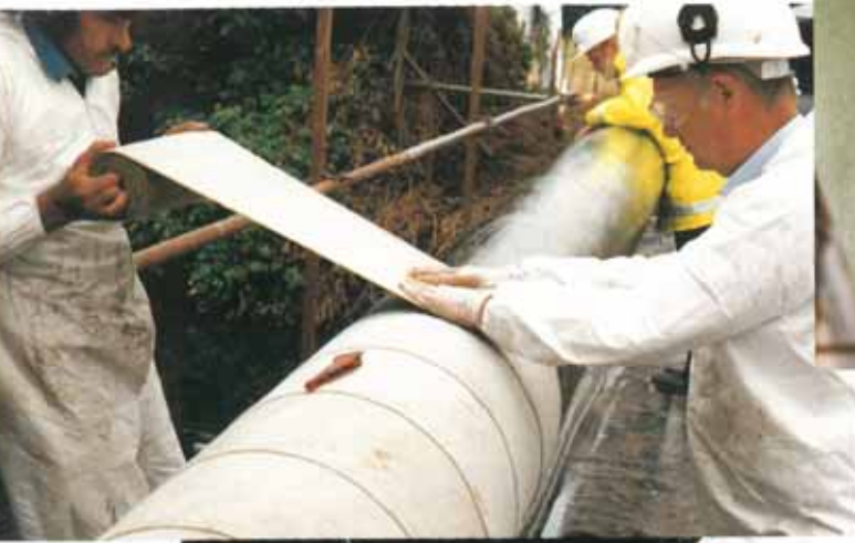
Denso Covercoat Tape is applied to pipe.
