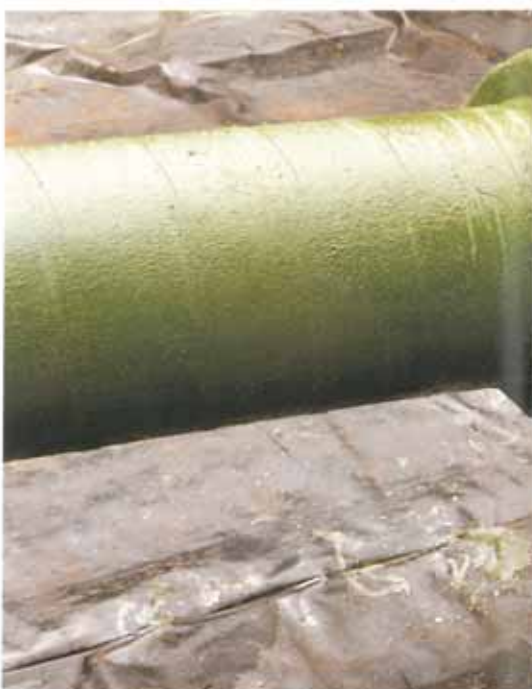
Denso Profiling Mastic is used to build up joints prior to wrapping.
