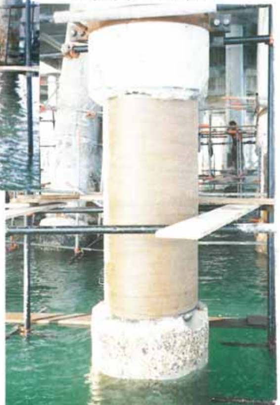
A completed pile prior to concrete replacement.
