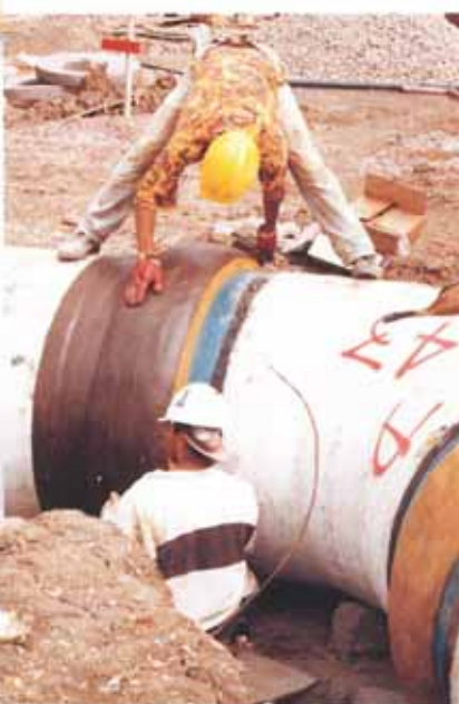
Denso Polythene Cling Wrap completes the system.
