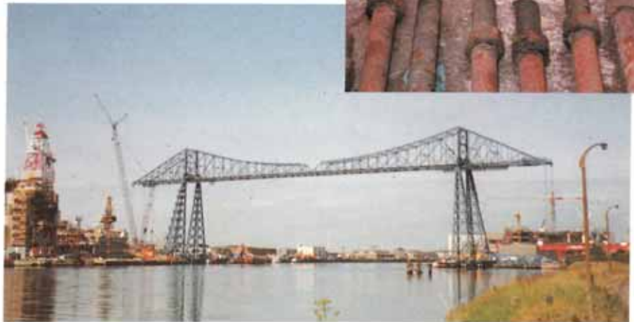
The transporter bridge.
