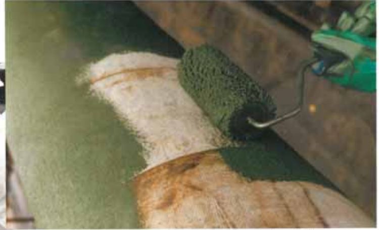
Covercoat Epoxy Compound can be applied by roller.
