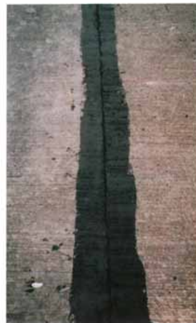
Tokseal Primer applied to joint in carriageway.
