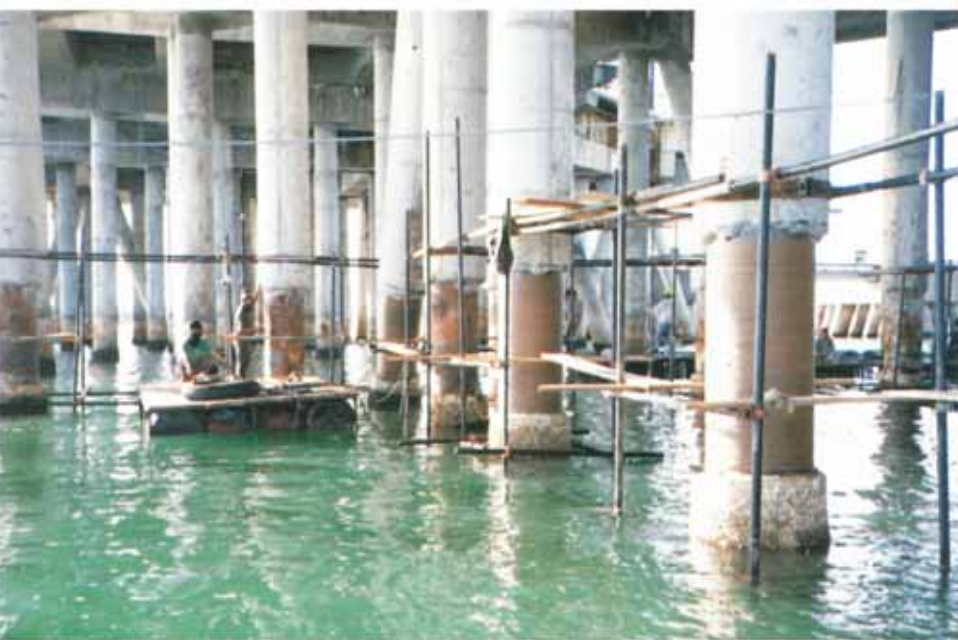
The Seashield system at various stages of completion:
