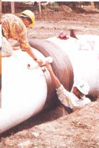
Denso Polythene Cling Wrap completes the system.
