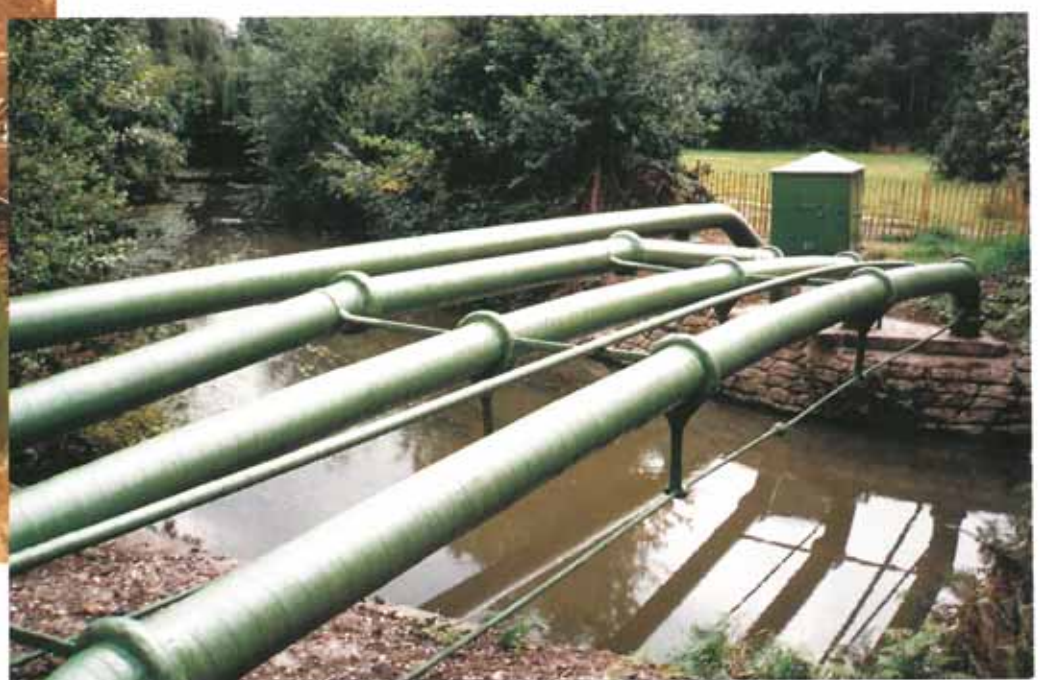
Covercoat Epoxy Compound, brush applied to mechanical joints.
