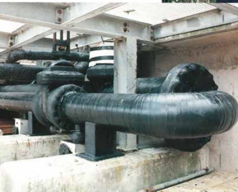
Above: Denso Tape overwrapped with Densoclad 40.
