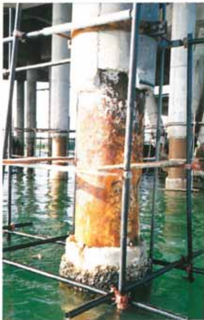
After removal of the concrete the steel surface was cleaned.
