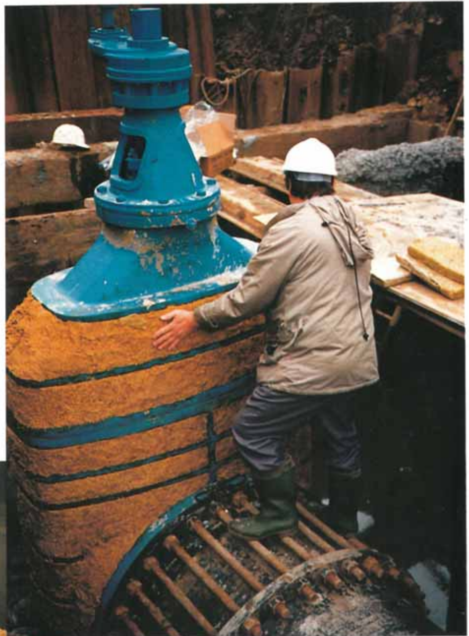
Denso Profiling Mastic applied to a valve.
