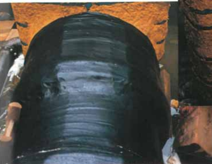
Densoclad 40 applied over Denso Profiling Mastic.
