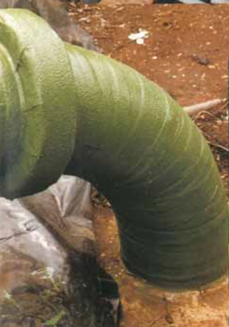
Covercoat Epoxy Compound, brush applied to mechanical joints.
