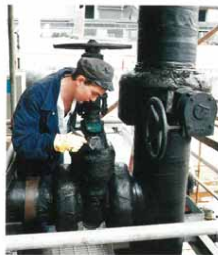
Solvent free epoxy Denso Covercoat gives a tough finish.
