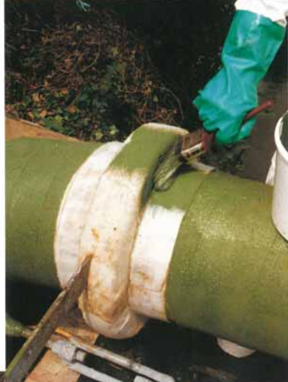
Covercoat Epoxy Compound, brush applied to mechanical joints.
