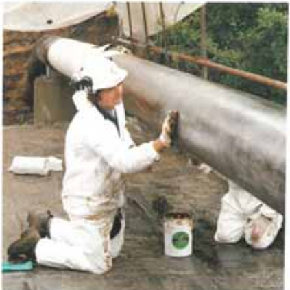
Application of Denso Priming Paste.
