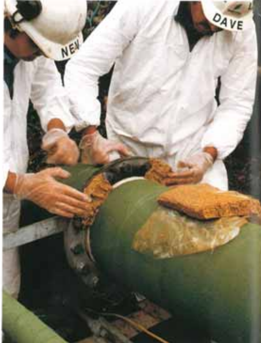
Denso Profiling Mastic is used to build up joints prior to wrapping.
