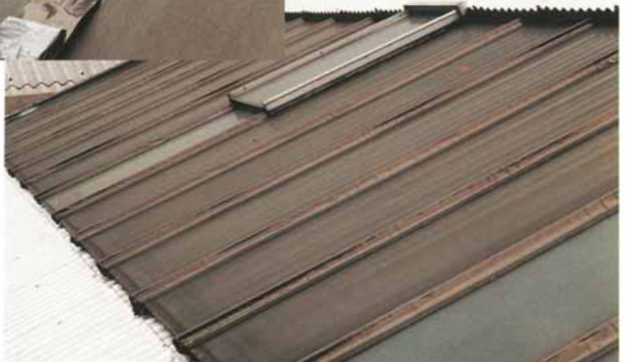
A finished section showing weatherproofed glazing bars.
