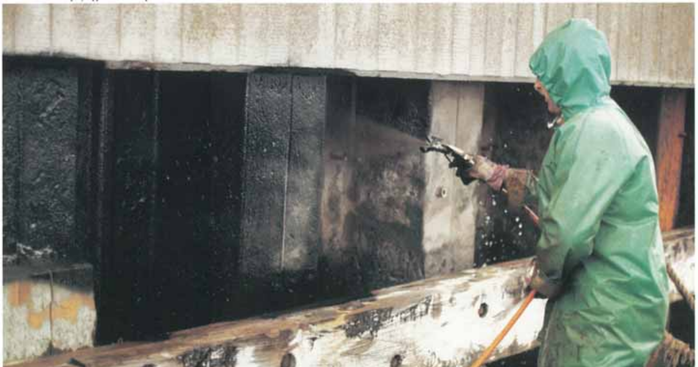
Denso Protal 5065 spray applied to tidal/splash area.
