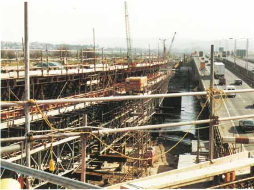
Construction underway on the relief scheme alongside the M4 motorway.
