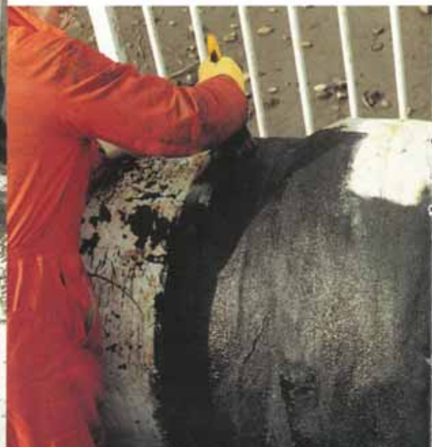
The first coat of Denso Covercoat Epoxy Compound is applied to the Covercoat Tape.
