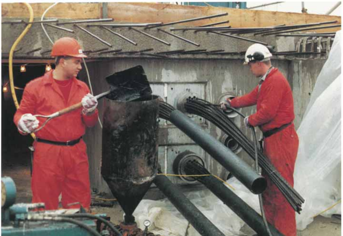
Denso Void Filler applied to the stressing cable tendons.
