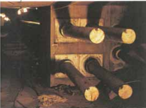
The ends of the tendons are capped off to allow easy access for monitoring their condition.
