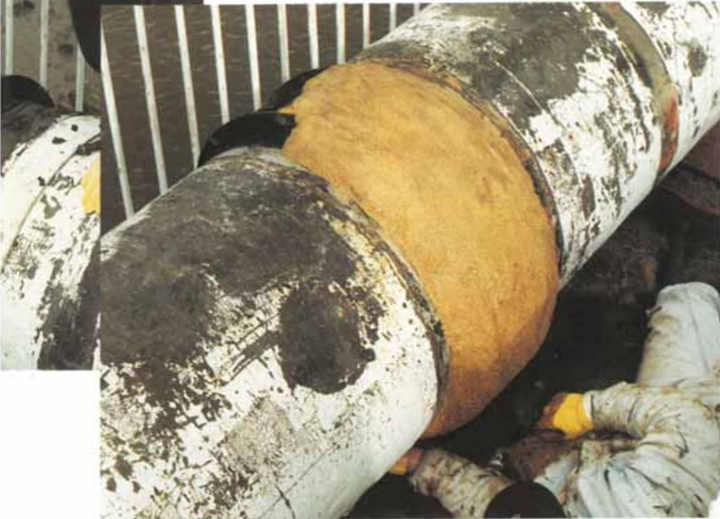
The joint profile is built up using Denso Profiling Mastic.
