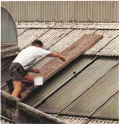
Application of Denso Flashing Tape Primer.
