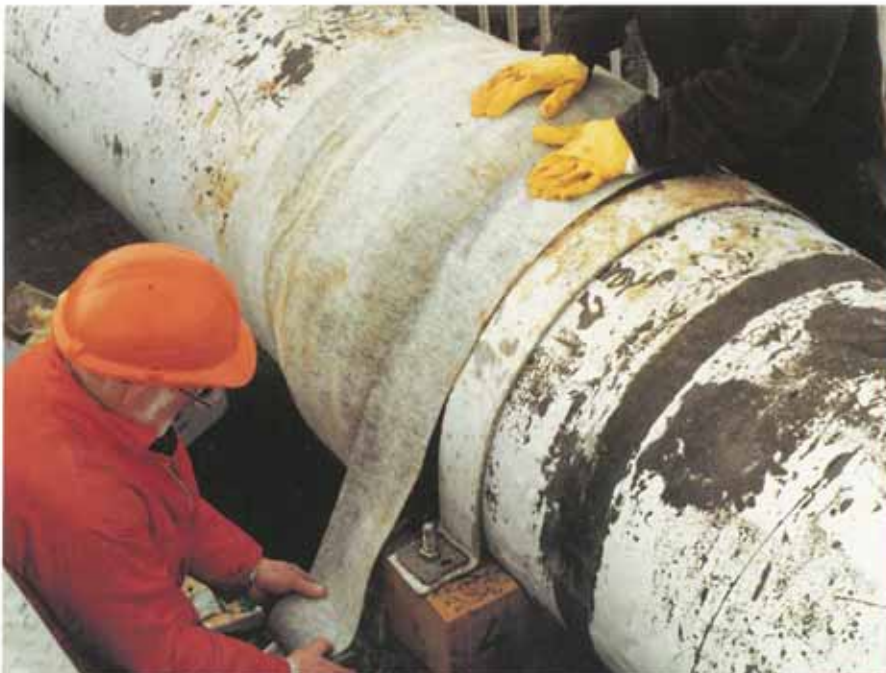
The first coat of Denso Covercoat Epoxy Compound is applied to the Covercoat Tape.
