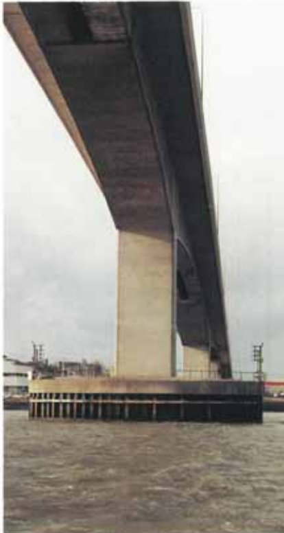
One of the bridge supports.
