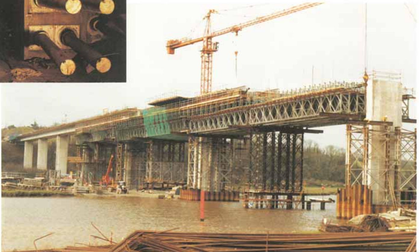
The new road bridge during early stages of construction.
