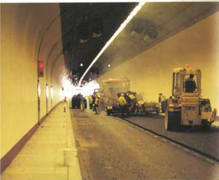
The wearing course is laid up to the Tokband Spezial.
