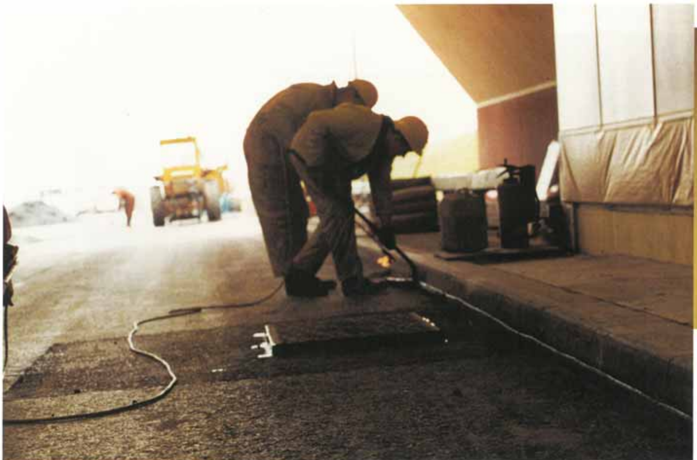
Application of Tokband Spezial to kerb edge.
