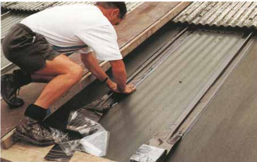
Denso Flashing Tape applied to the primed glazing bars.
