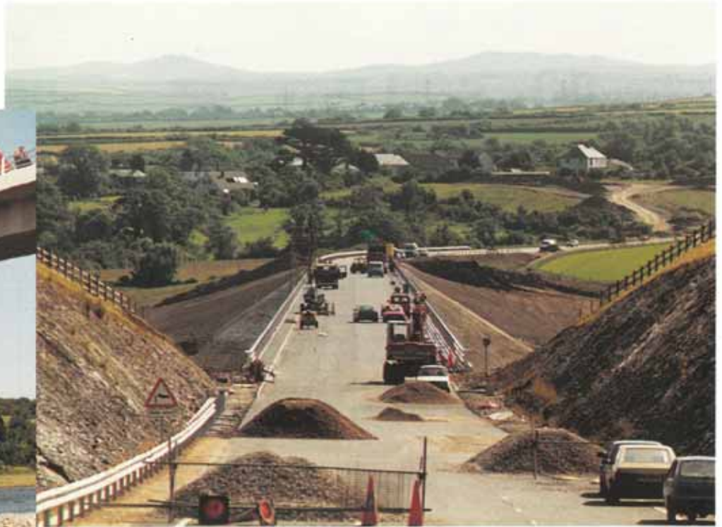
View over top of new road bridge.
