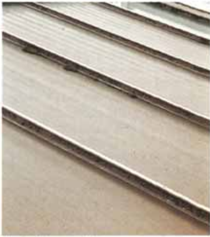
The glazing bars prior to cleaning.
