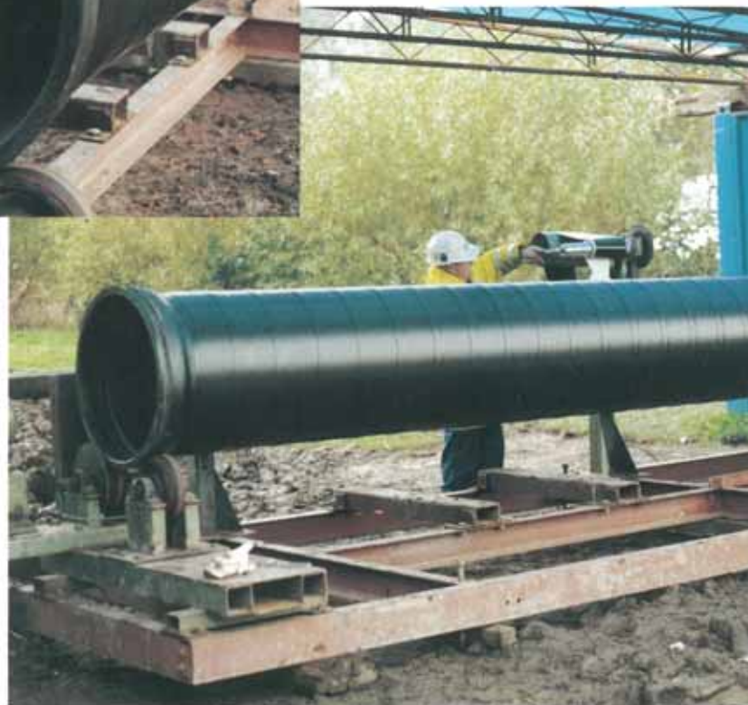
Rolling rig application of Densoclad 70S Tape underway.
