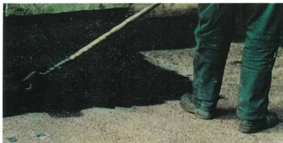
Denso Drive Refurbisher is applied by roller.
