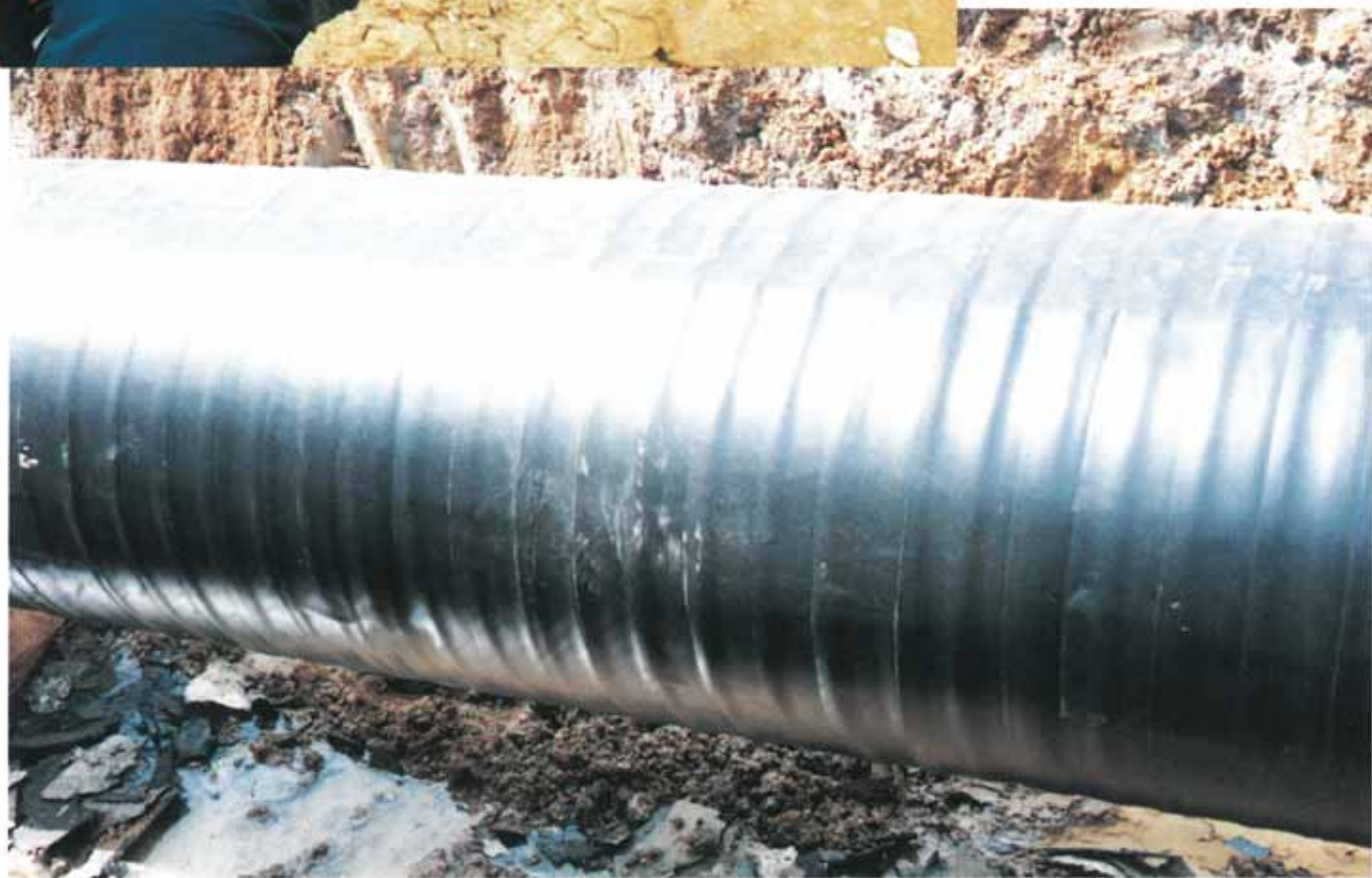
The Demosem Wrapping Machine gives a tight, uniform tape application.
