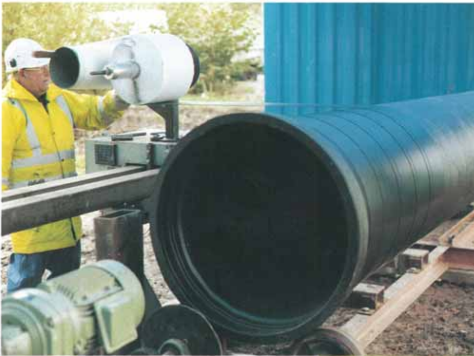
Rolling rig application of Densoclad 70S Tape underway.
