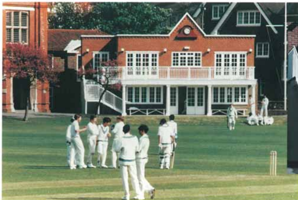
The R.G.Howell Memorial Pavilion with Protal coated staircase and balcony.
