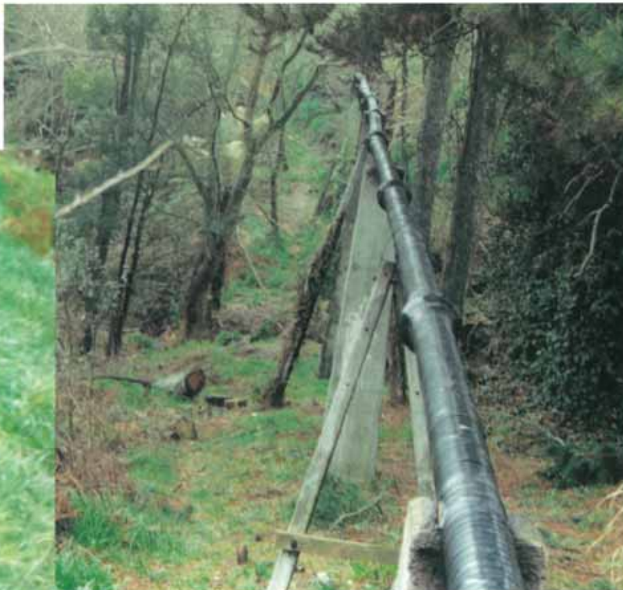
The protected domestic sewer line.
