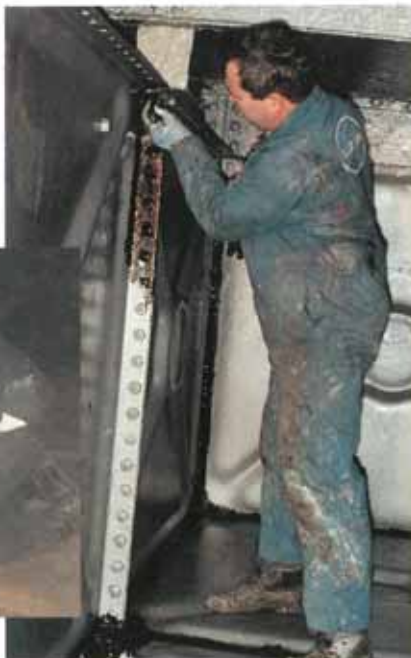
Application of stripe coat to edges and external angles.
