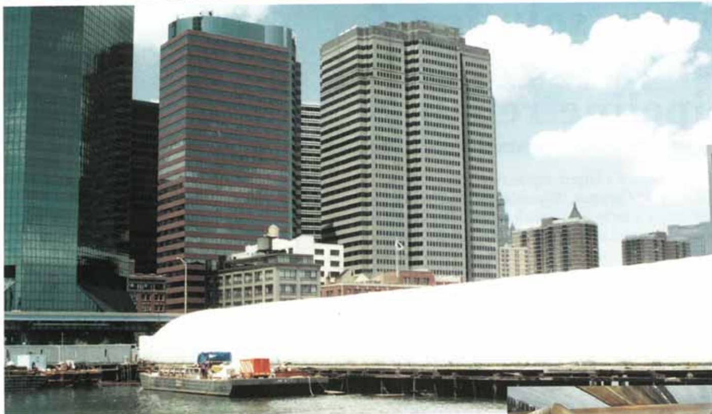
The SeaShield Series 40 System was used to protect timber piles of Piers 13 & 14 at the New York Health & Racquet Club.
