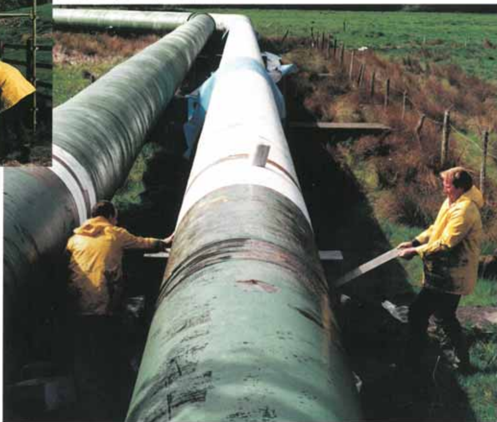
Application of Denso Covercoat Tape
