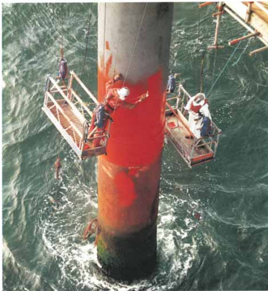
Spray application of Rigspray.
