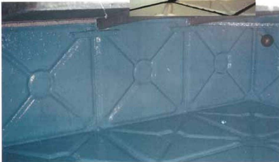
Final application of Nu-Tank 400E topcoat (blue).
