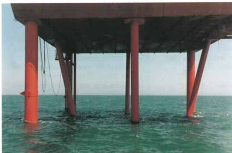
Sections of oil rig riser protection frames coated with Archco-Rigidon Rigspray material for Amoco.
