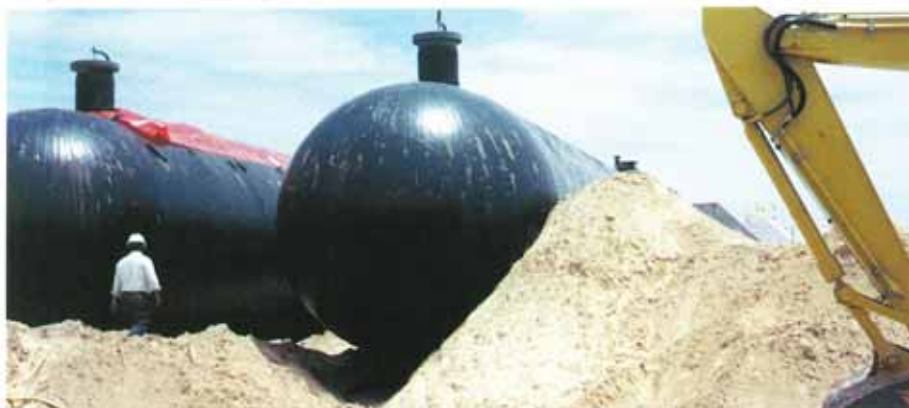
Burying Bullets with fine washed sand, required 8000 tonnes.
