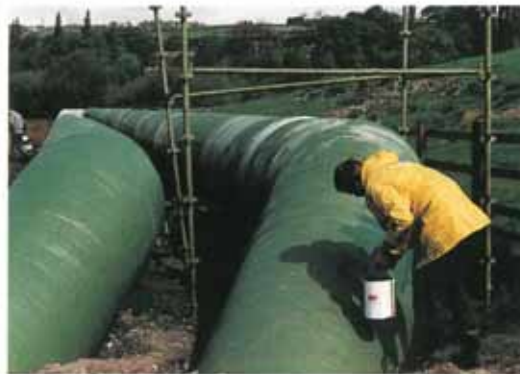
Denso Solvent-free Epoxy Coating is easily applied by brush.
