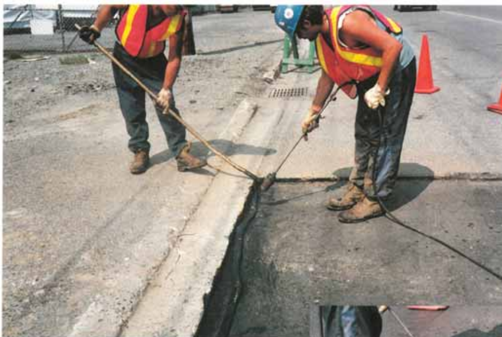
Tokband Spezial used to form an effective seal between a concrete curb and an asphalt reinstatement
