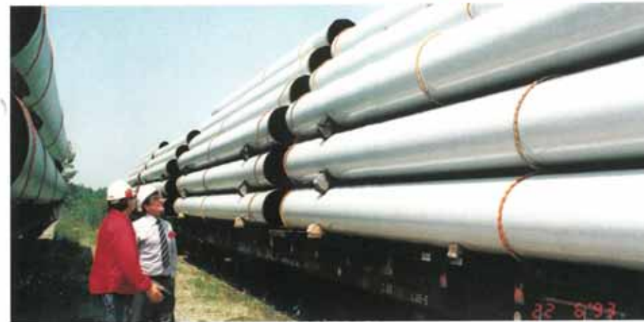
12m x 1.06m (40' x 42") lengths of steel pipe for road and river crossings protected by Protal 5900 over F.B.E. mill coating ready for rail transportation to job site.
