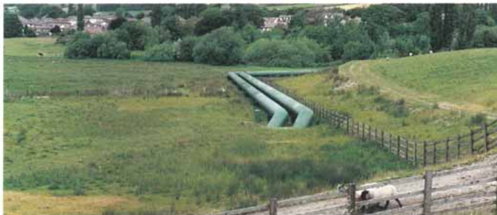
The completed Denso Covercoat System
