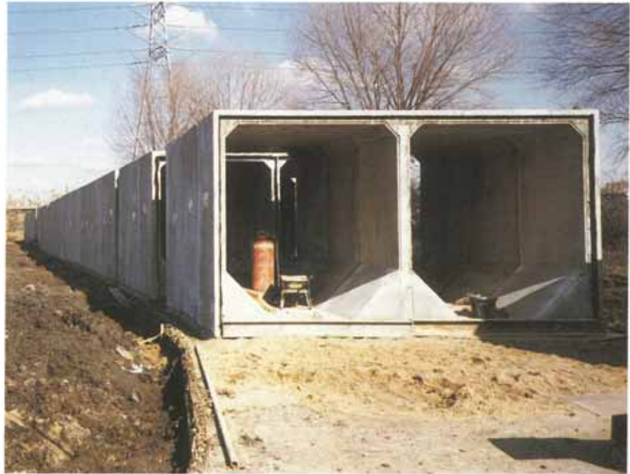
Twin cell concrete box culverts specially designed by FC Precast Concrete of Derby.
