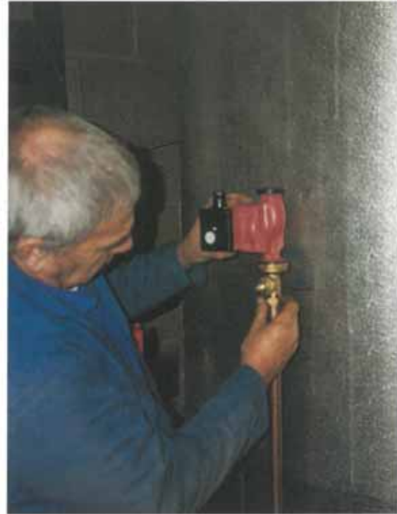
Installing a destratification pump.
