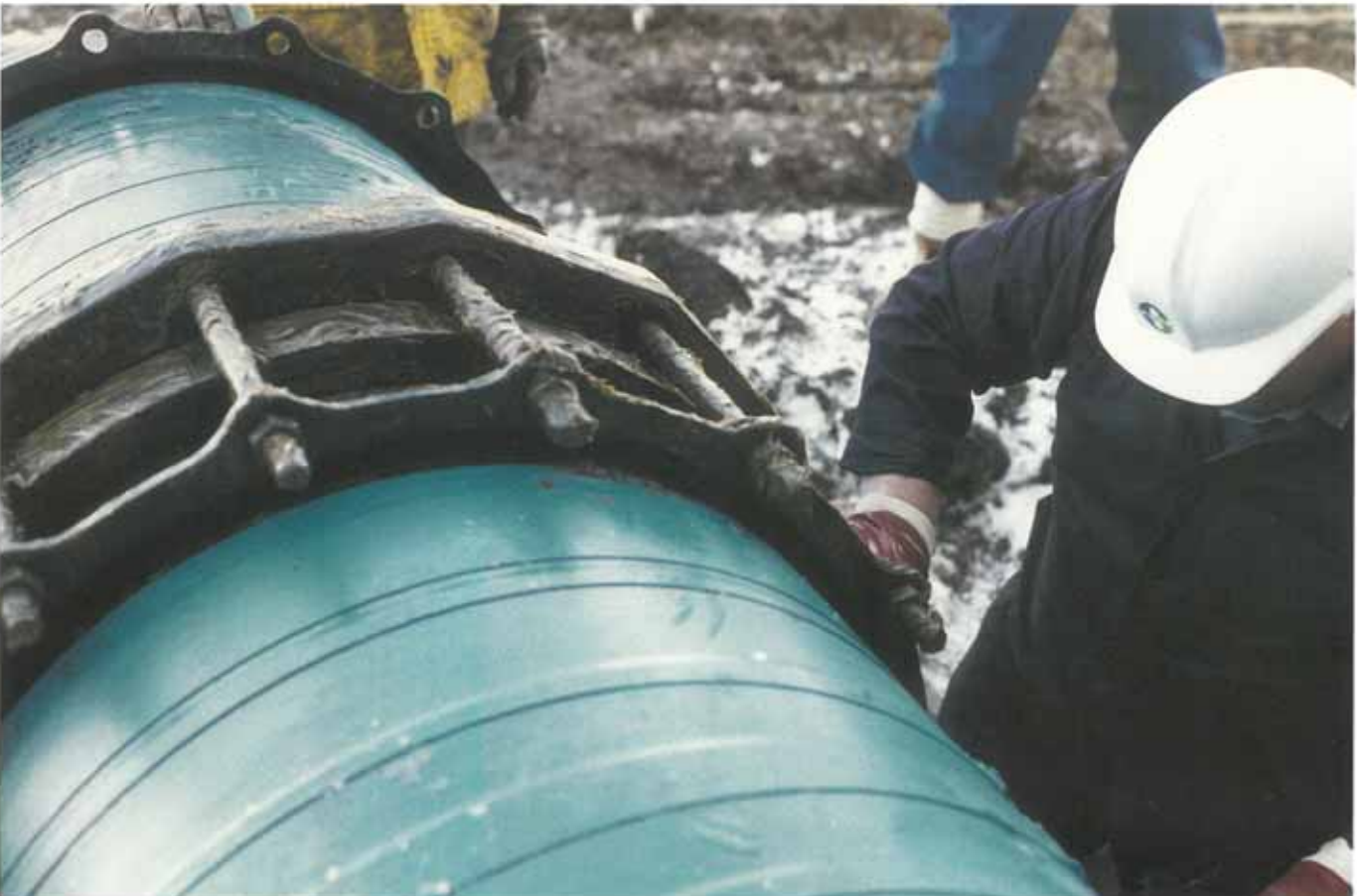
Denso Paste applied to Tybar joint.
