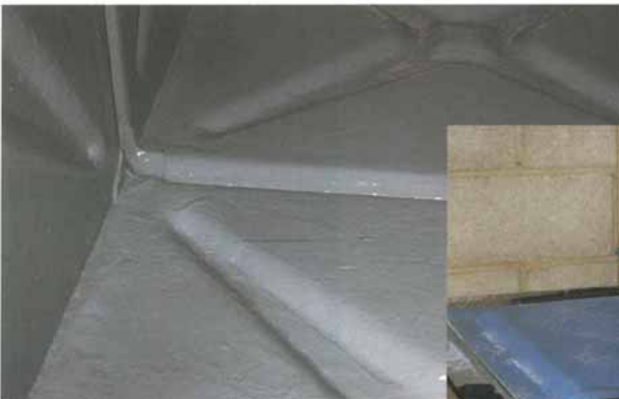
Tank re-lined with Nu-Tank 400E.
