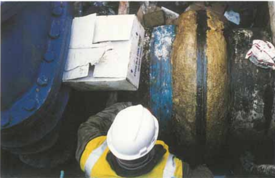
Denso Profiling Mastic is used to smooth the joint's contours.
