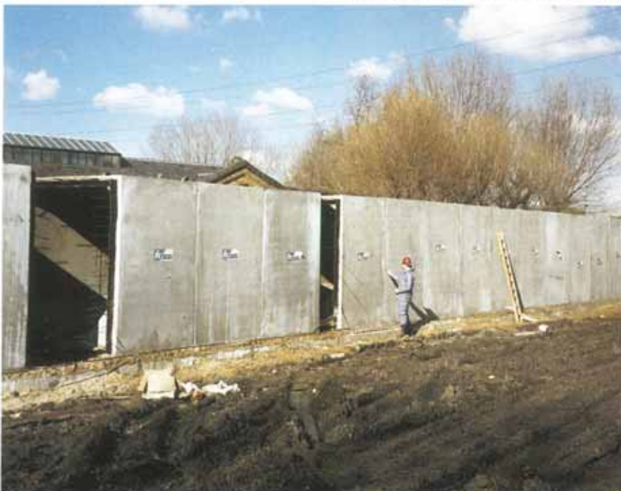
Culverts installed with Tokstrip used as the joint sealant.
