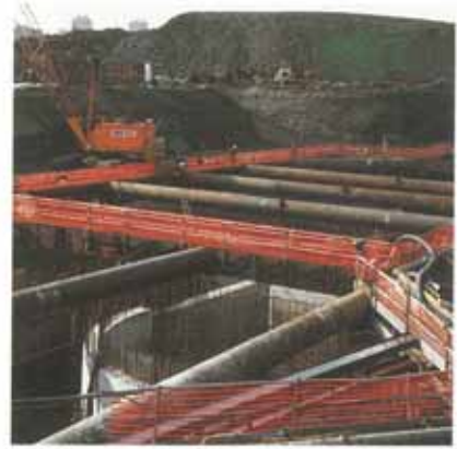
The Abbey Mills development site.
