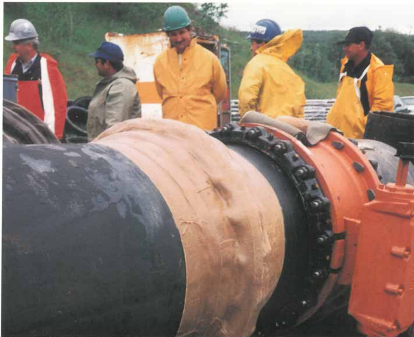
Water main joint protected with the specified Denso system.
