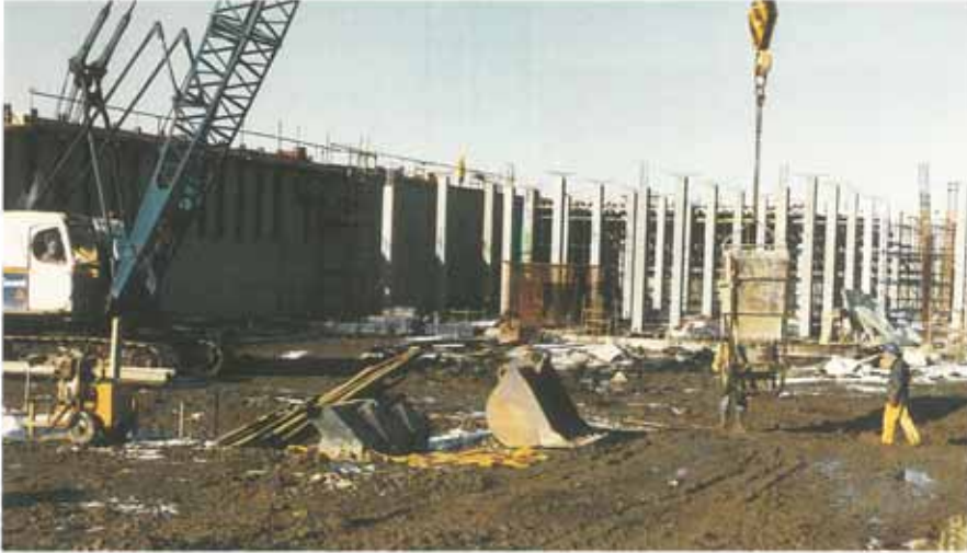
The new reservoir during construction.
