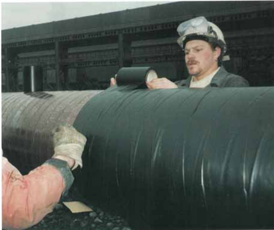
The Denso machine gives even tension and maintains the correct overlap for wrapping pipelengths.
