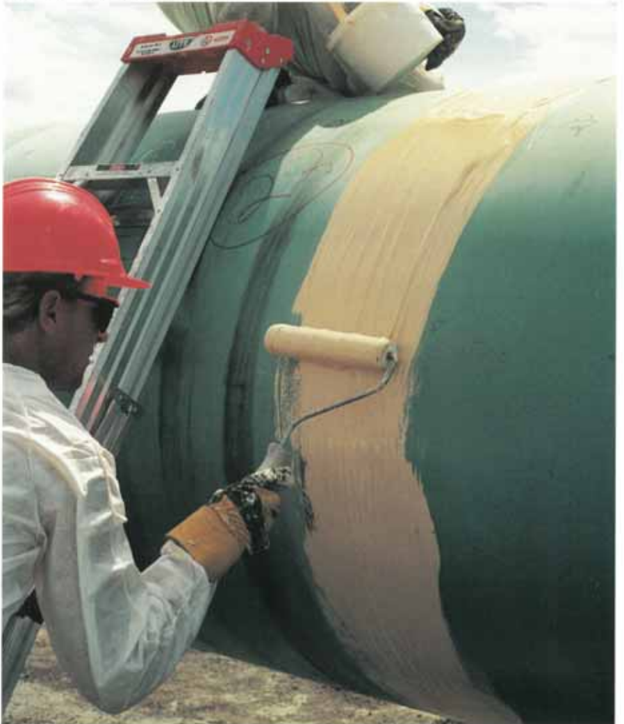
Application of Protal 7000 by roller.
