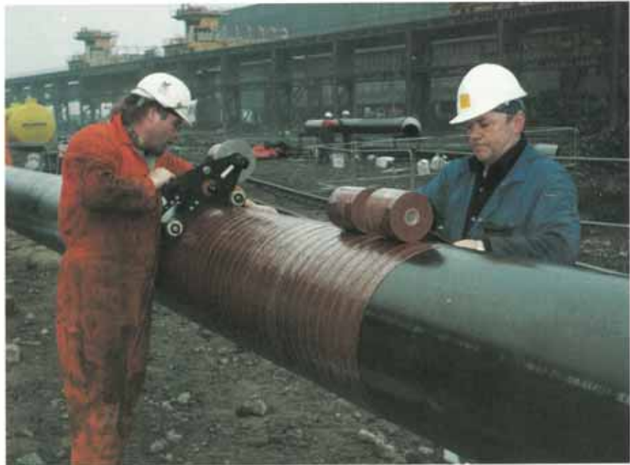
The Denso machine gives even tension and maintains the correct overlap for wrapping pipelengths.
