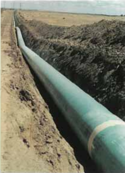
Protal 7000 application to a girth weld.
