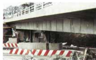
The A31/A3 bridge at Guildford
