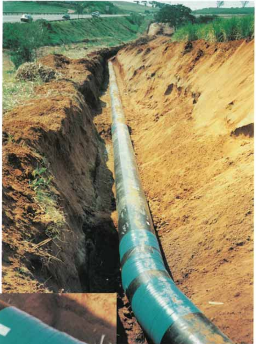
Denso Ultraflex Tape is ideal for the protection of butt welded joints, bends and fittings.
