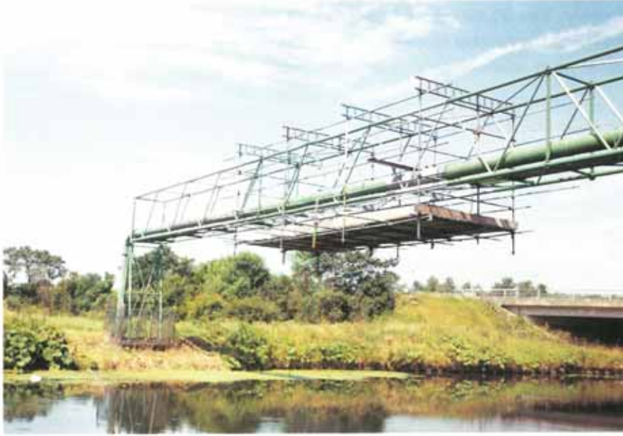
Transco gas main and bridge structure over the River Ancholme protected with the Denso Steelcoat system.
