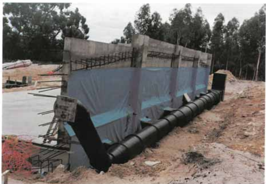
Air conditioning duct work protected with the Densopol 60 System.
