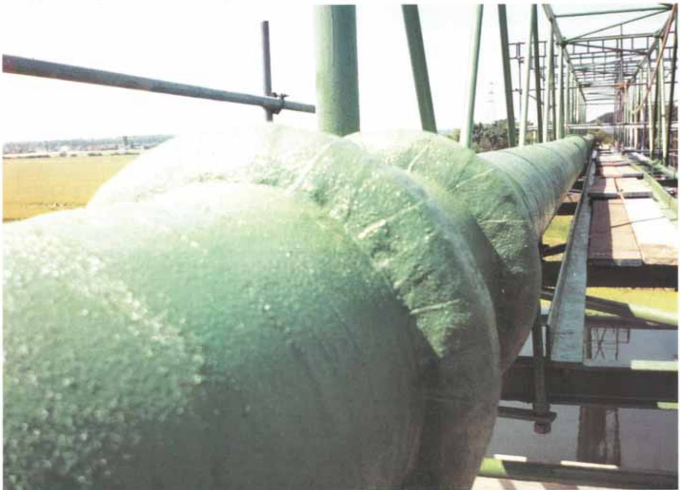
Transco gas main and bridge structure over the River Ancholme protected with the Denso Steelcoat system.
