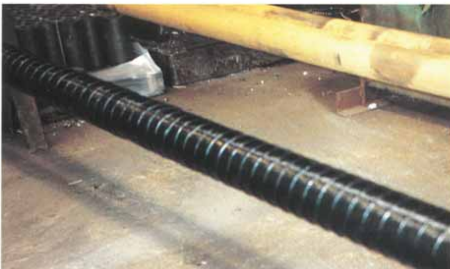
Close up of a protected tie-bar.
