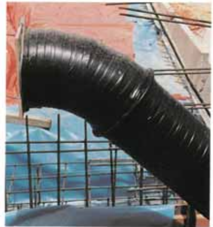
Air conditioning duct work protected with the Densopol 60 System.
