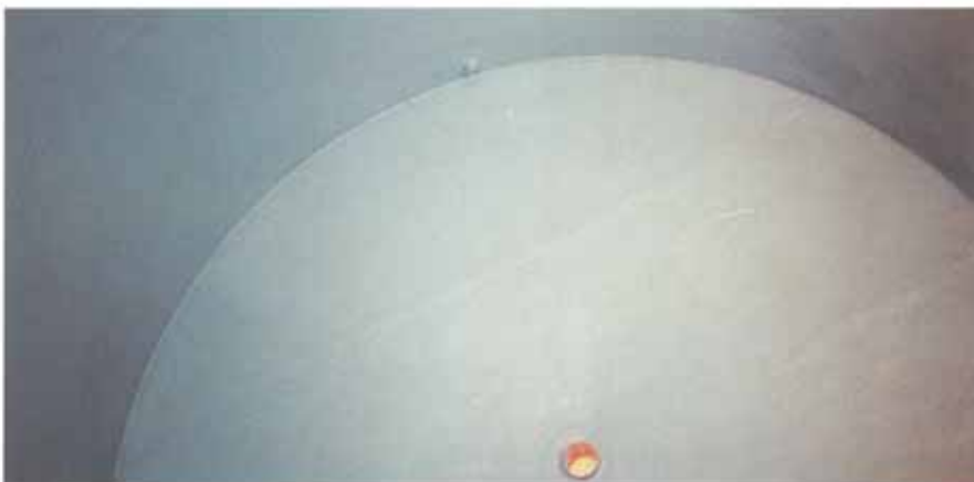
Close-up of completed tank lining.
