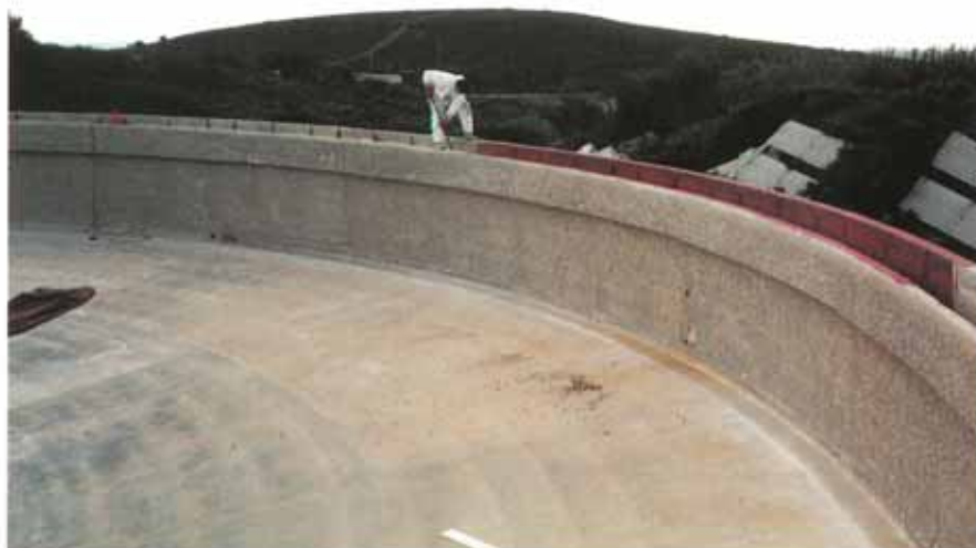
Application of the lining in progress.
