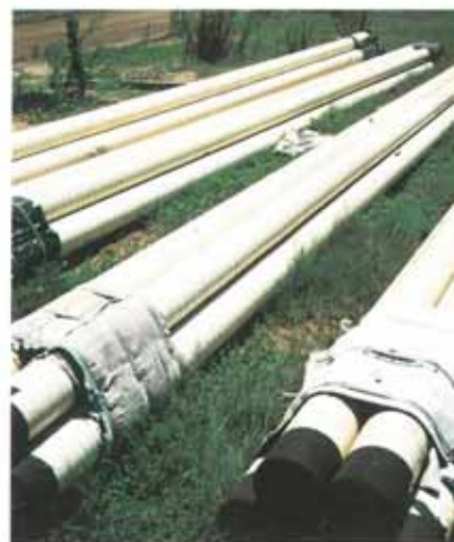
Denso Ultraflex Tape wrapped pipelengths ready for installation.
