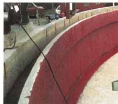
The finished lining will protect the concrete from attack by the acids and alkalis present in the clay slurry.
