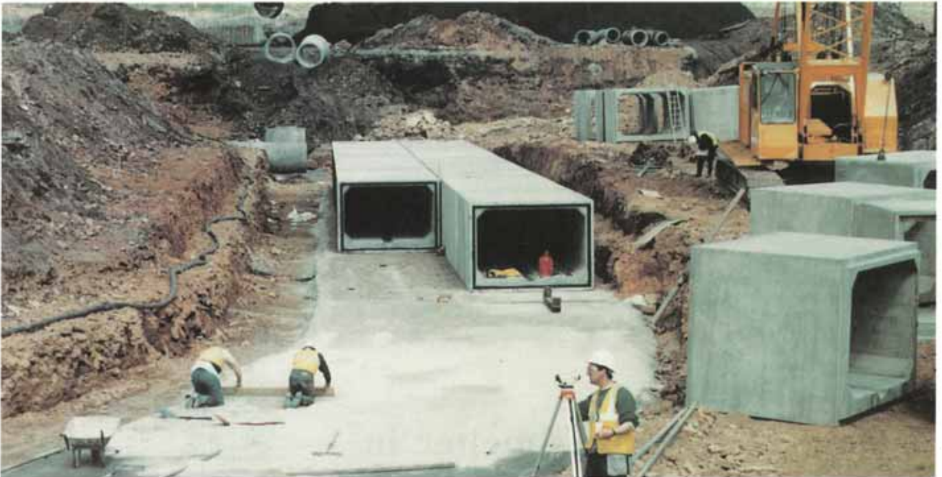
The first few Uniflow box culverts in position jointed with Tokstrip.
