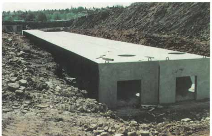
The water storage tank nears completion.
