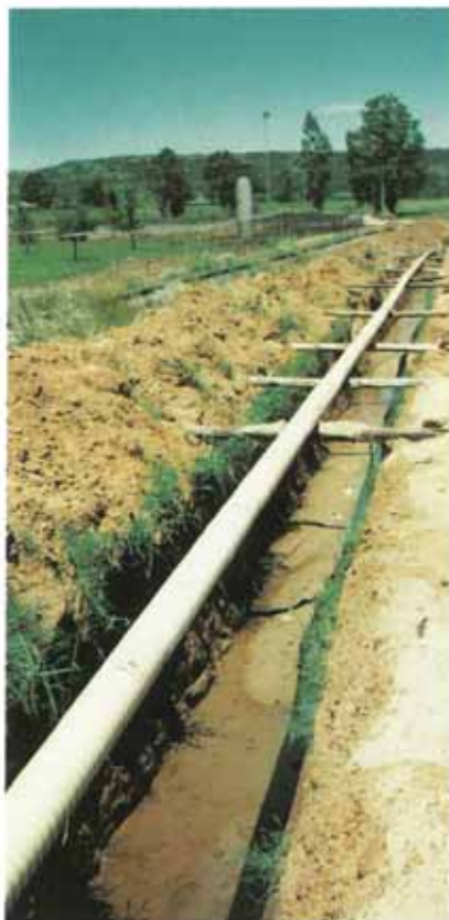
The Denso protected oxygen pipeline under construction.
