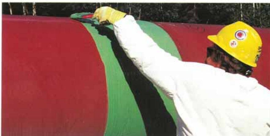
The coatings can be brush, roller or spray applied.
