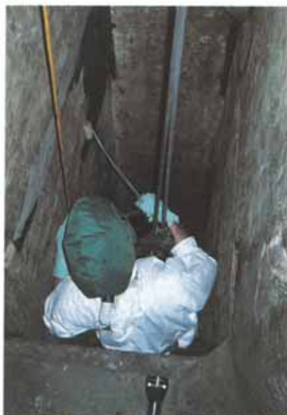
Application of Denso S.T. Epoxy to the riser shaft.
