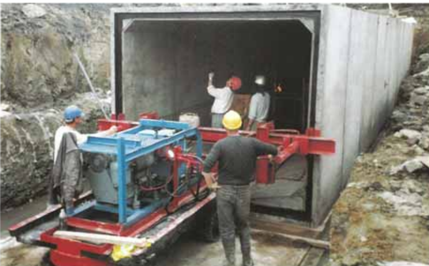
Box culvert units jointed with Tokstrip.
