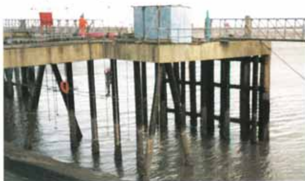
One of the dolphins undergoing renovation.
