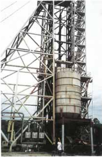
The Cargill Salt steel head frame.
