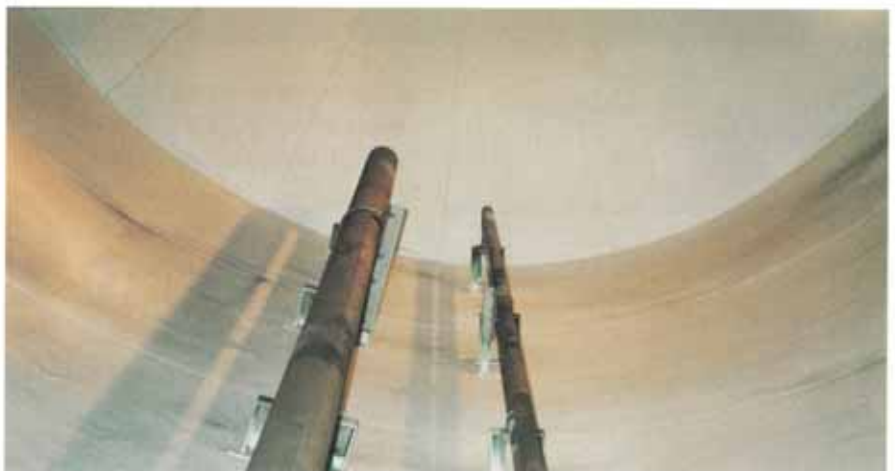
Below: Internal view of the completed Archco-Rigidon system
