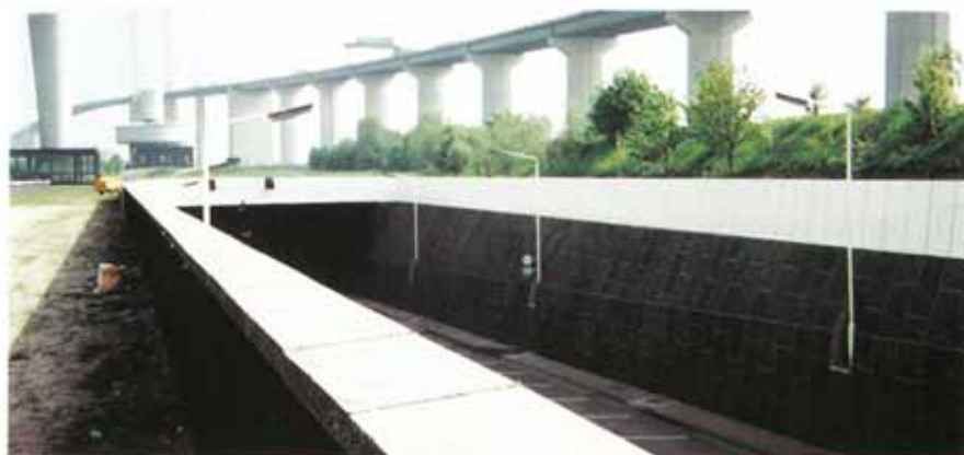
The Dartford East Tunnel entrance.
