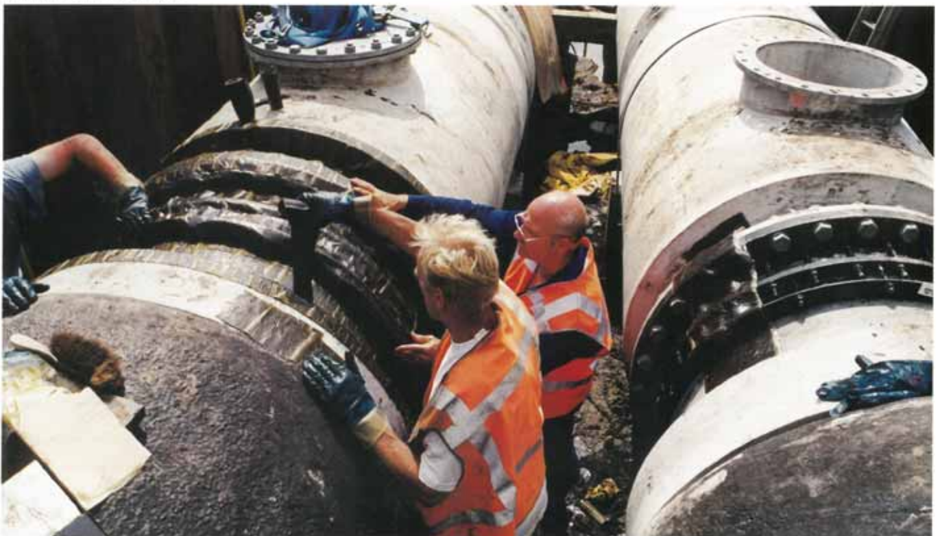
Application of the Denso Tape system.
