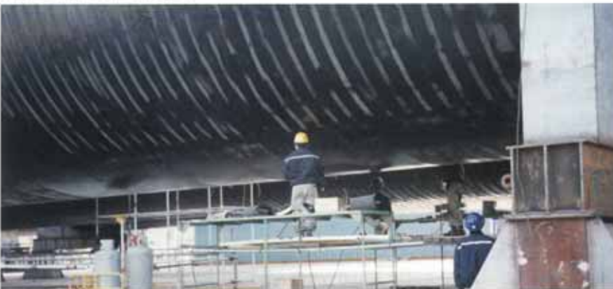
Above: Wrapping the tanks with Densotherm 35 Tape.
