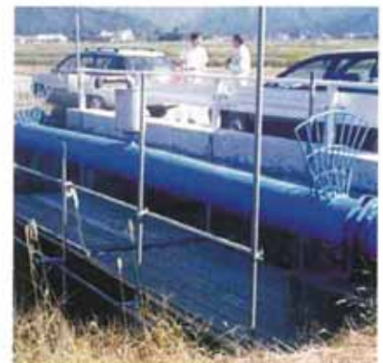
Above: The protected water pipebridge.
