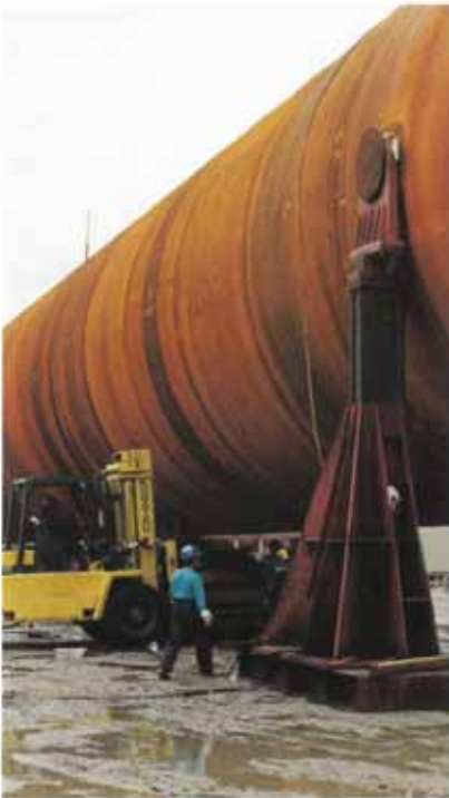
The tanks were first cleaned to SA2½.
