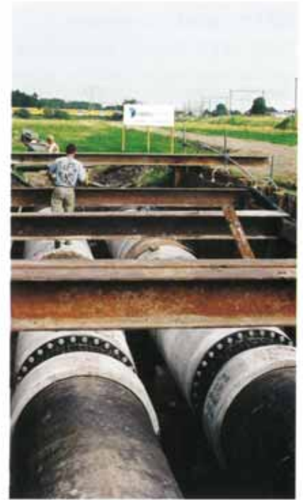
Two of the rehabilitated pipeline's VJ couplings ready for Denso protection.
