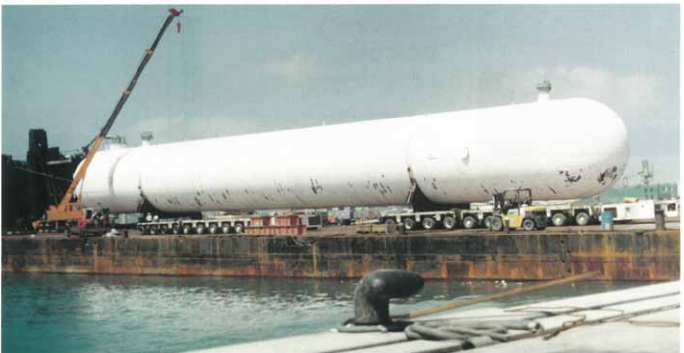
Below: The finished tanks were blinded with white water based coating to reflect the sunlight during transportation.
