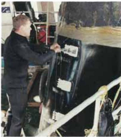
Application of the SeaShield 2000 System.
