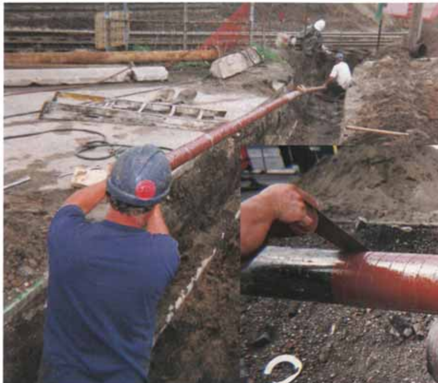
Above: Installation of the new high temperature edible oil pipelines.
