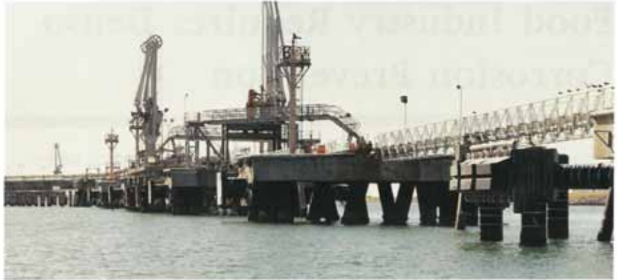
The Arco Pipeline Dock.
