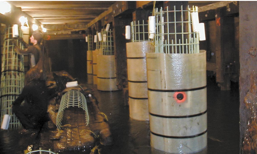
Above: The SeaShield Fiber Forms are positioned around the timber piles. Below: Completed SeaShield Fiber-Form system.
