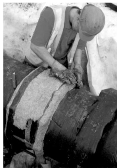
Denso Profiling Mastic was used to smooth the profile of the couplings prior to wrapping with Densoclad 70 Tape
