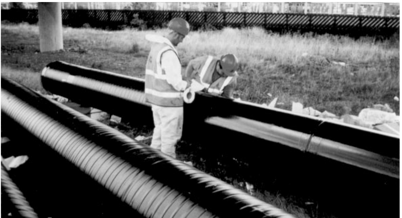
The Pipelengths being wrapped with Densoclad 70 Tape.
