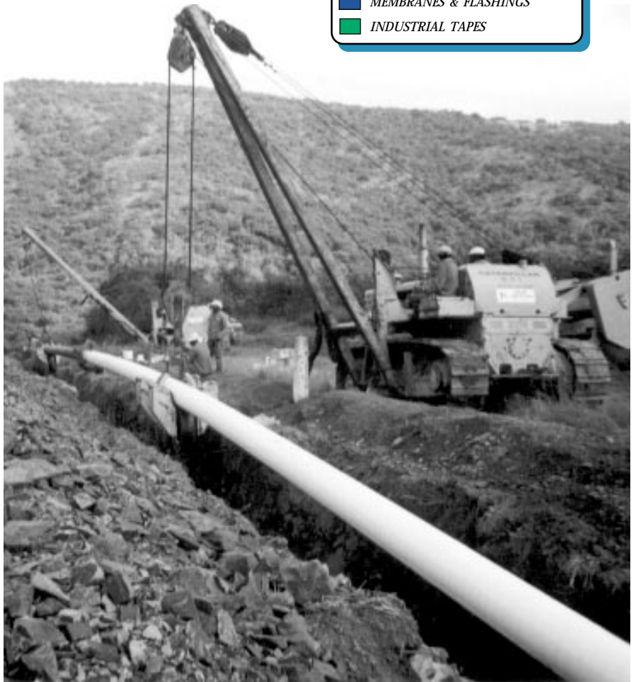
Above: The Denso system is applied prior to the pipe being 'snaked' into the trench.
