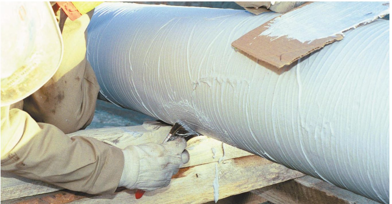
Below: Protal 7125 is applied by brush at pipe support areas that were left during roller application.
