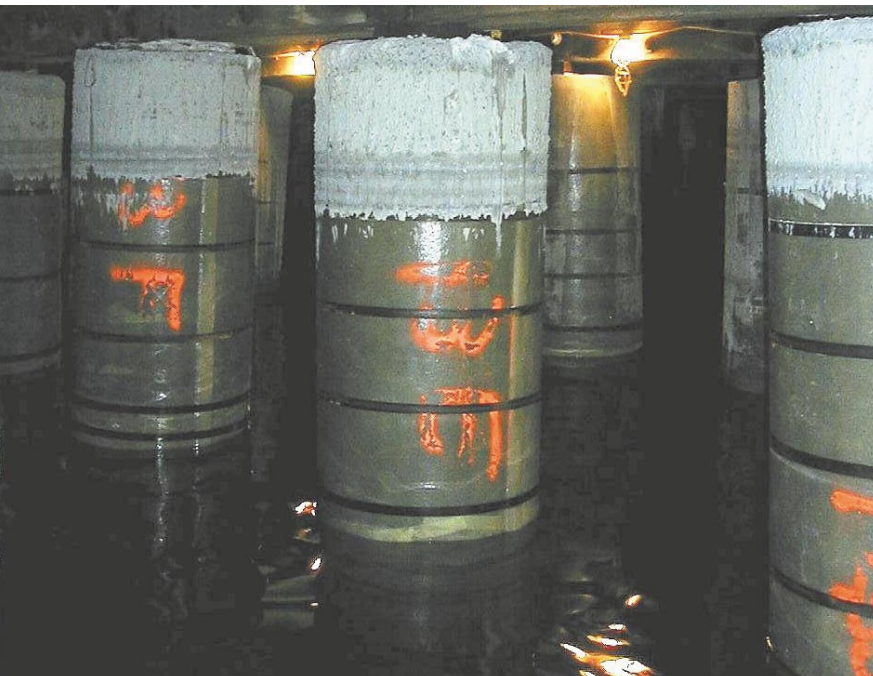
Above: The SeaShield Fiber Forms are positioned around the timber piles. Below: Completed SeaShield Fiber-Form system.
