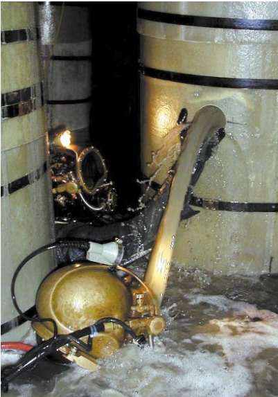
Above: Concrete is pumped into the annulus space between the jacket and timber pile.
