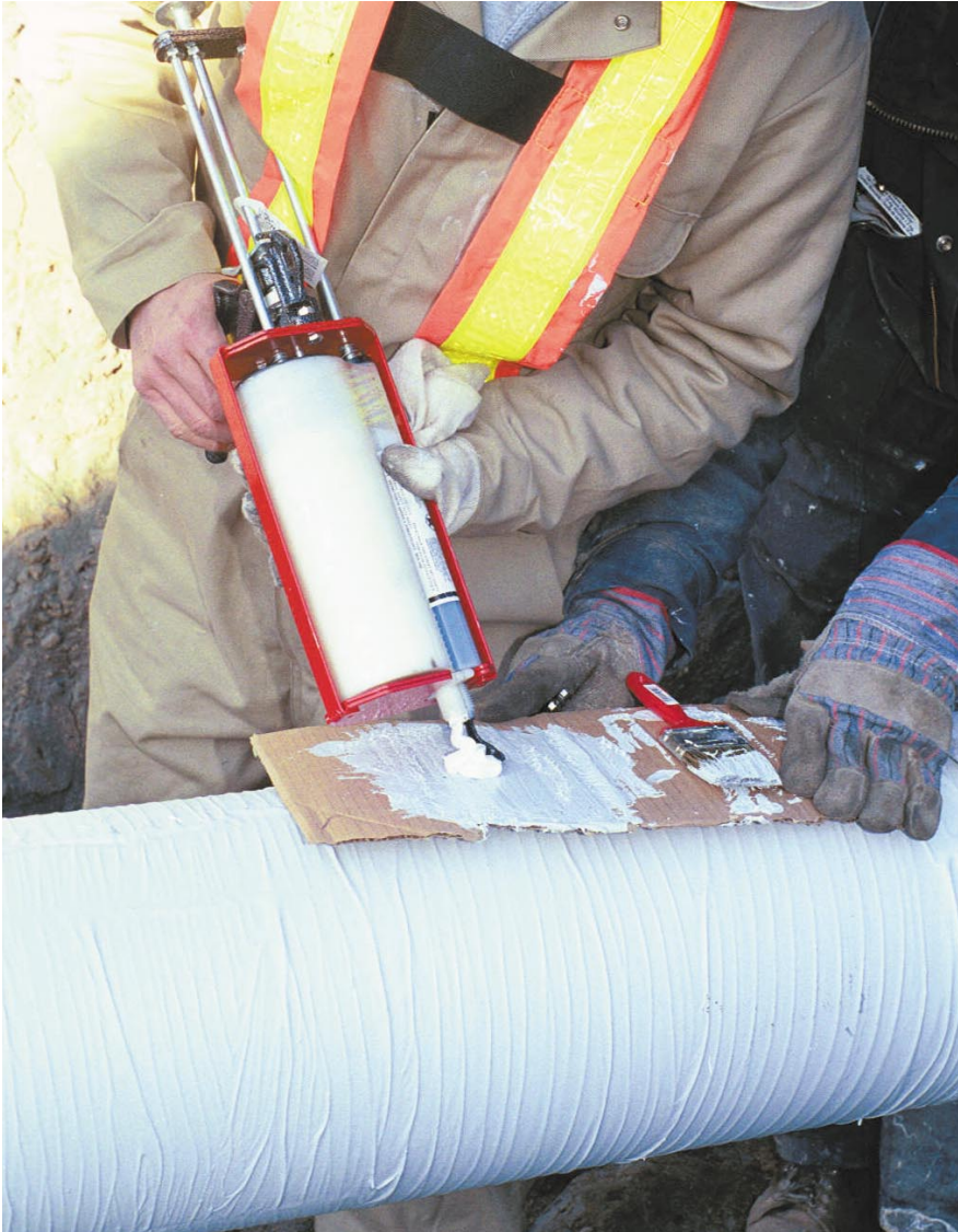
Above: Pipe coated with Protal 7125 that has been applied by roller. Protal 7125 Repair Cartridge being dispensed prior to mixing for brush application.
