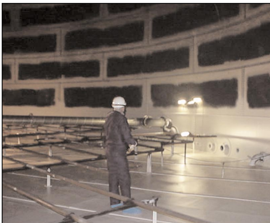
Work in progress inside the 1 \frac{3}{4} million gallon tank.
