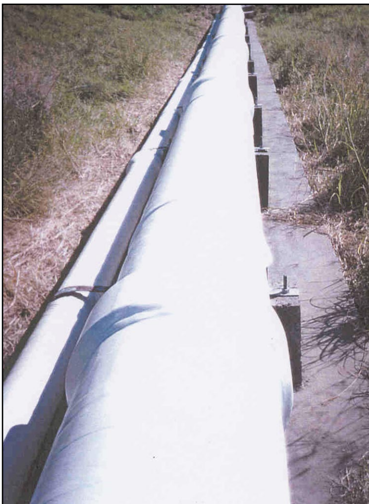
Above: The application of Denso White Colourtape.
