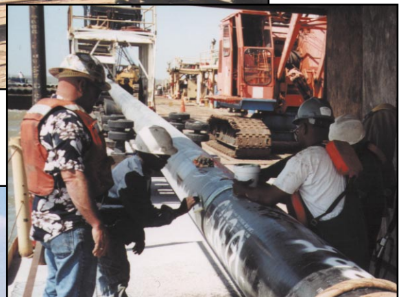
Below: Protal 7200 applied on girth welds allows the contractor to backfill quickly.
