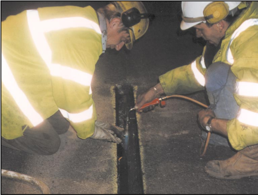
Densoband is applied vertically against the sound surface areas before infilling with Zebrascreed.
