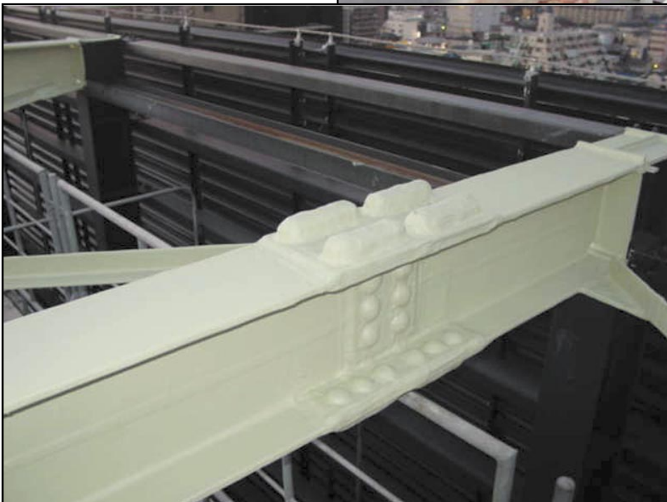
Above: The poor condition of the steelwork before grit blasting
