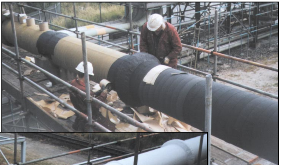
Above: Denso Ultraseal Tape is applied over the Denso Hi-Tack Tape.
