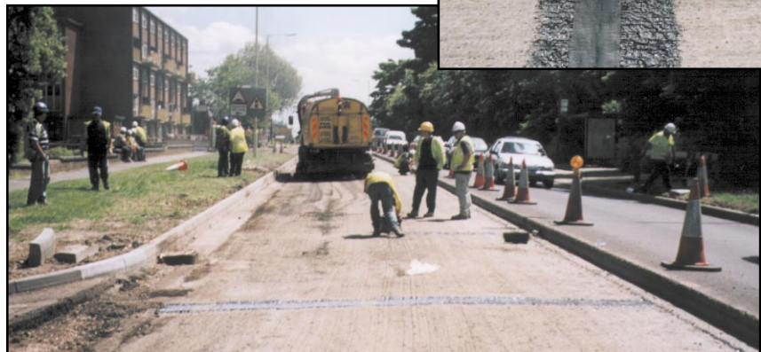
Denso Paving Tape is applied over the seams before overlaying with the asphalt base wearing course.
