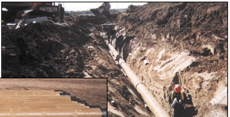
The pipelengths were wrapped outside the trench then lowered into position and joined together. The joints were then wrapped with Denso LT Tape.
