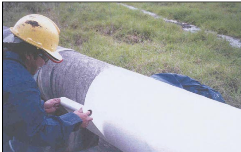
Above: The application of Denso White Colourtape.
