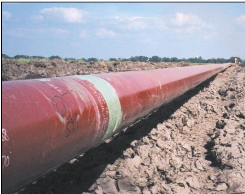
Below: Protal 7200 applied on girth welds allows the contractor to backfill quickly.
