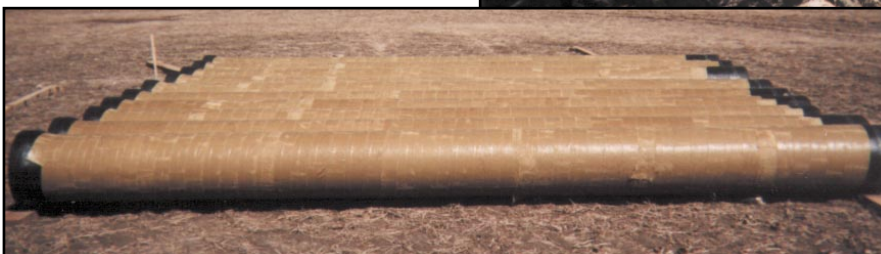
The pipelengths were wrapped outside the trench then lowered into position and joined together. The joints were then wrapped with Denso LT Tape.
