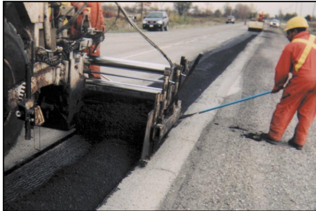
The new hot asphalt road surface is layed against the Densoband forming a waterproof seal.
