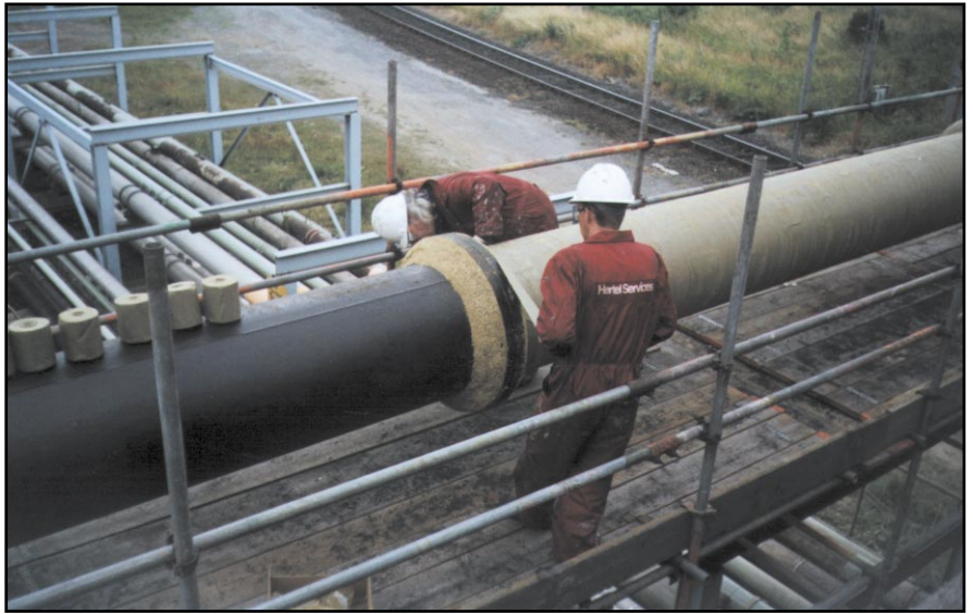
Below: Denso Hi-Tack Tape is applied over a coating of Denso Hi-Tack Primer.
