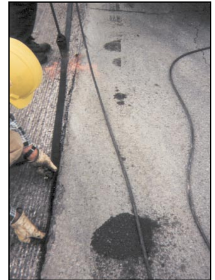
A Densoband jointing strip is positioned along the vertical face of a road joint.
