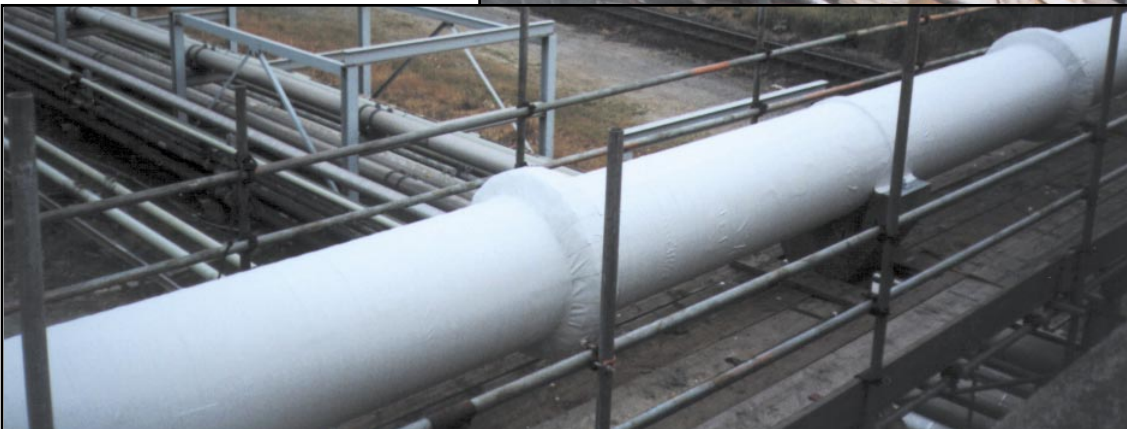
Above: Denso Ultraseal Tape is applied over the Denso Hi-Tack Tape.
