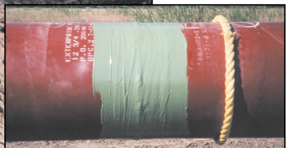
Above: The girth welds were coated with 25-30 mils of Protal 7200 in one coat.
