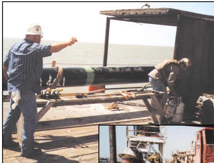
Below: Protal 7200 applied on girth welds allows the contractor to backfill quickly.
