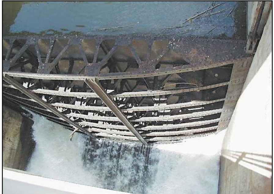
Above: A barrage gate in a partially lifted position clearly showing the water turbulence.
