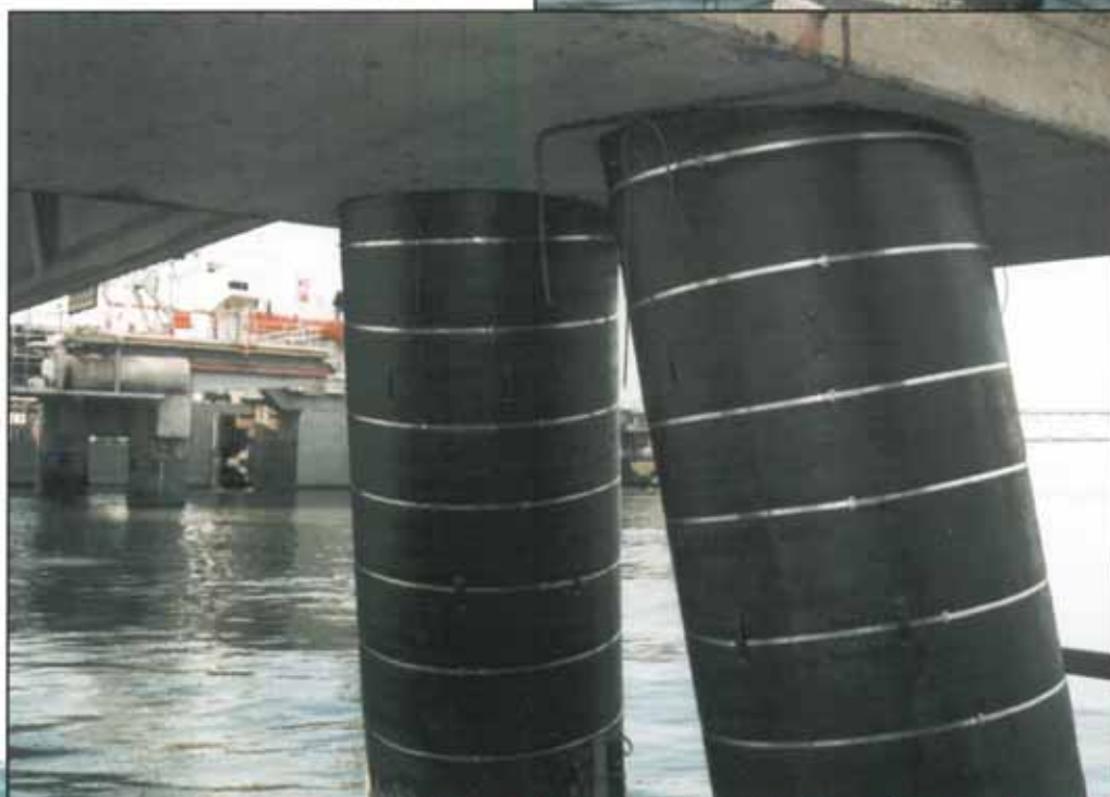
Above: SeaShield 100 Jackets being installed above the SeaShield 200 system.
