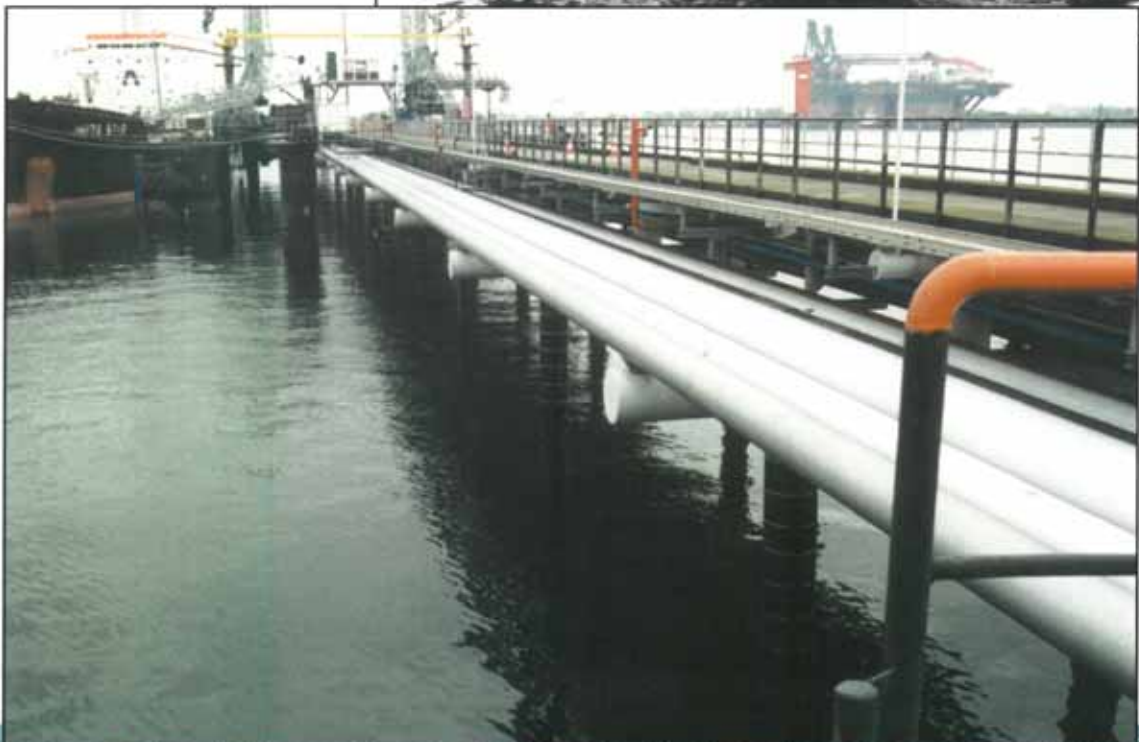
Right & Below: The completed installation of the SeaShield 100 system.
