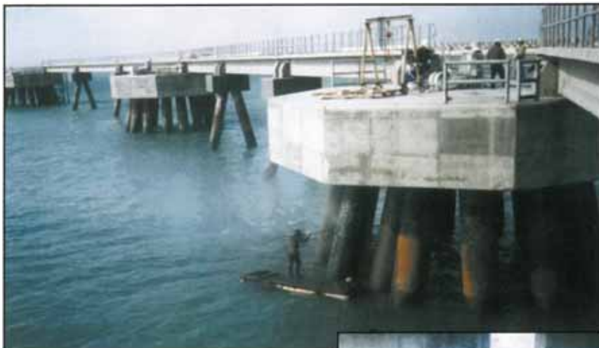
Above: High pressure water cleaning of the pile.
