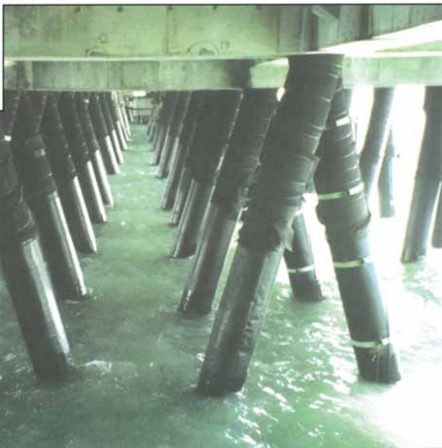
Below: Lower section of the piles protected with SeaShield 200 system.
