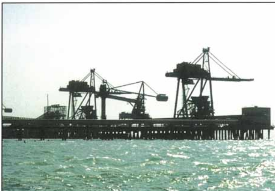
Above: View of the Hong Kong Electric Co. Ltd jetty.
