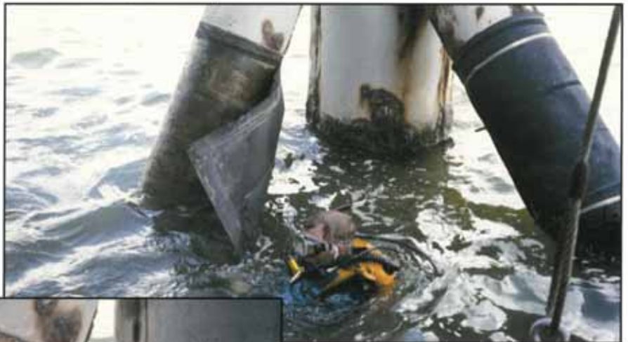
Above: Removal of the SeaShield Jackets.
