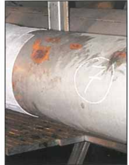
Above: There is no need for grit blasting when using the surface tolerant Denso Steelcoat 300 System.
