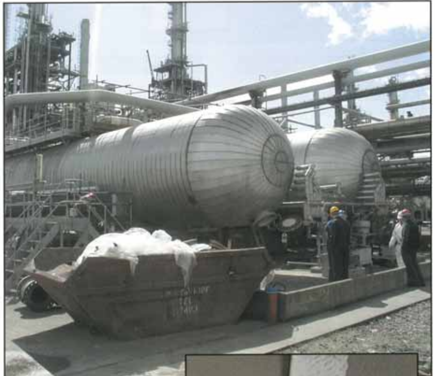
Above: The two desalter vessels at the North Sea Oil Terminal, Seal Sands near Middlesborough.
