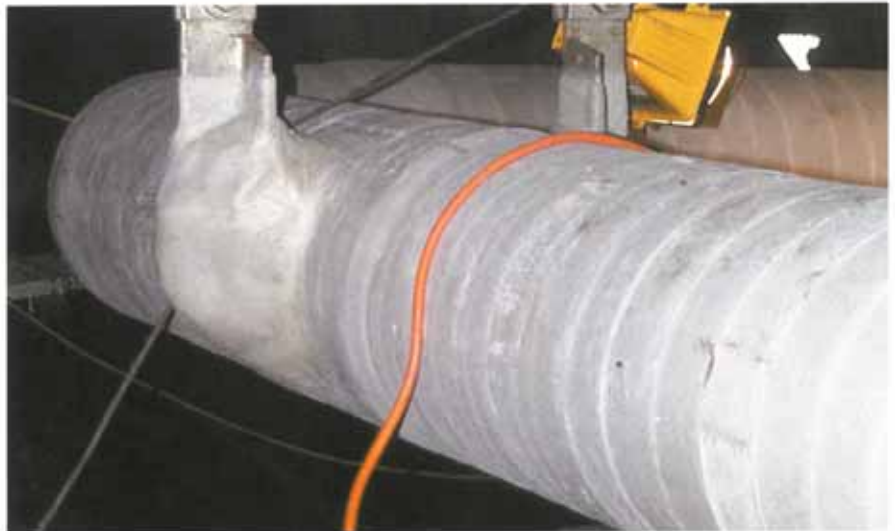
Above: There is no need for grit blasting when using the surface tolerant Denso Steelcoat 300 System.
