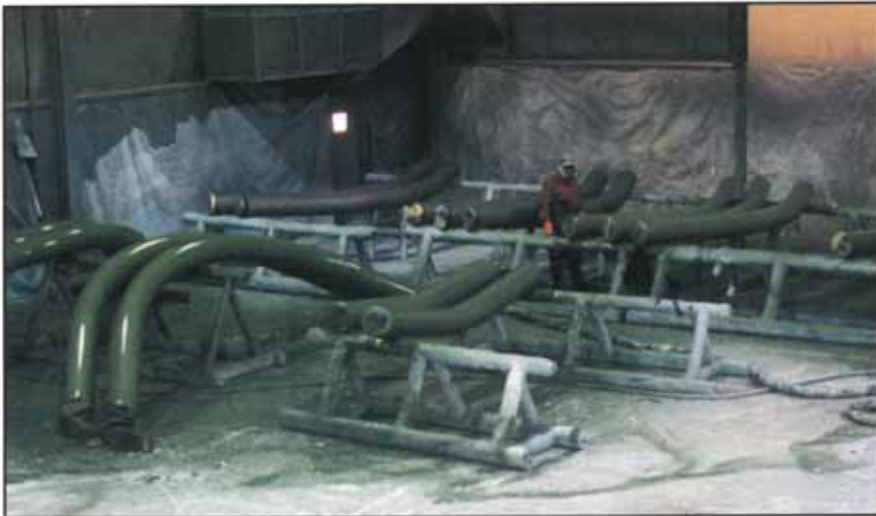
Protal 7250 spray applied to pipelengths in the shop.
