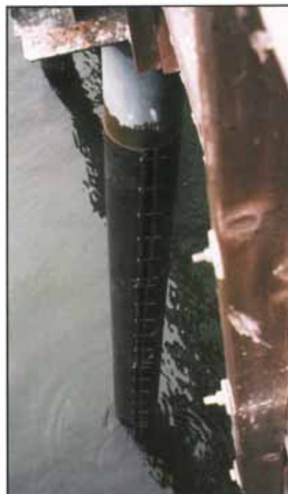
Above: The completed SeaShield Series 2000HD showing the fastener strip and marine grade 316 stainless steel bolts.
