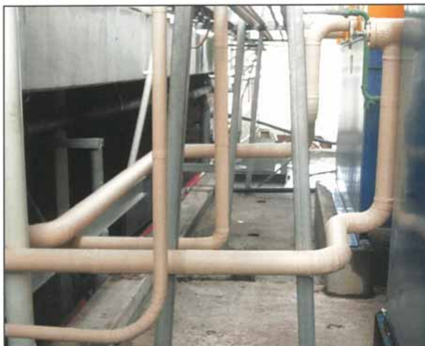
Above and below: Denso Steelcoat 400 protects the exposed process pipework at Darling Downs Bacon.
