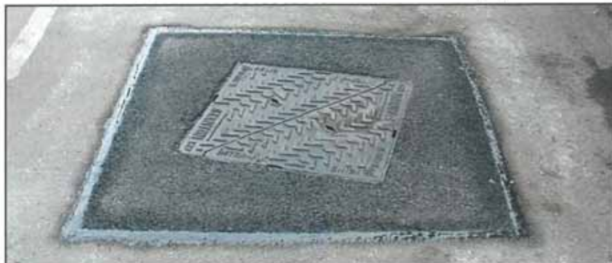
One of the Denso Overbanding Tape sealed reinstatements.
