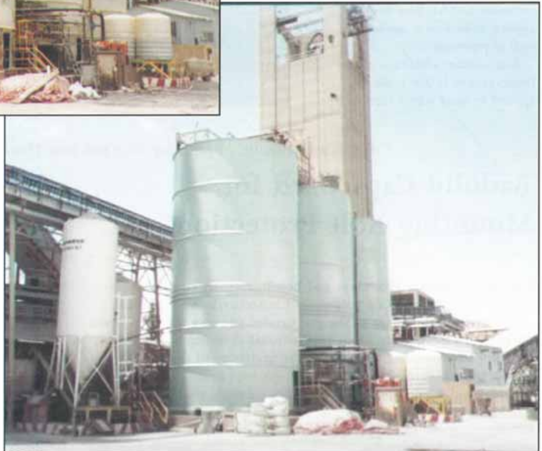
Above: The tanks after hand tool cleaning only.
