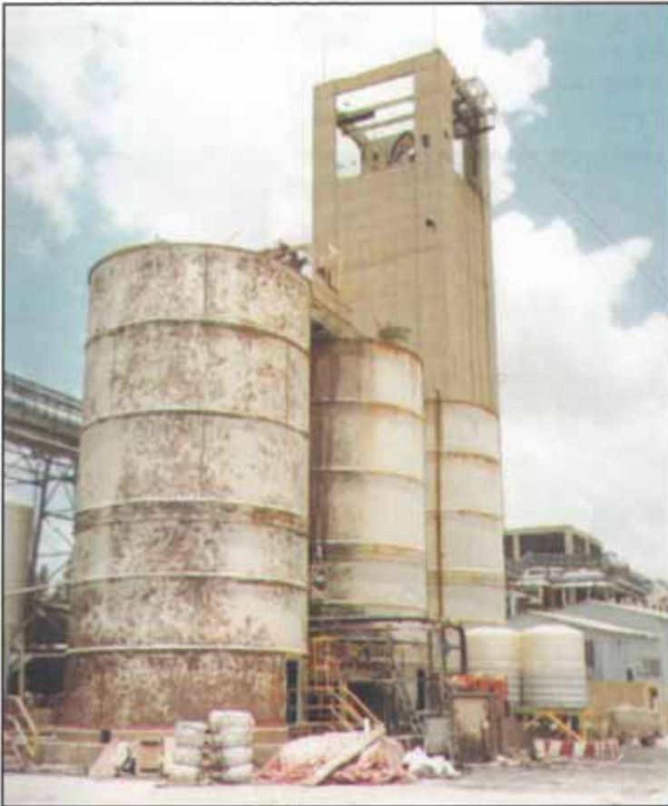
Above: The tanks after hand tool cleaning only.
