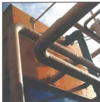
Above and below: Denso Steelcoat 400 protects the exposed process pipework at Darling Downs Bacon.
