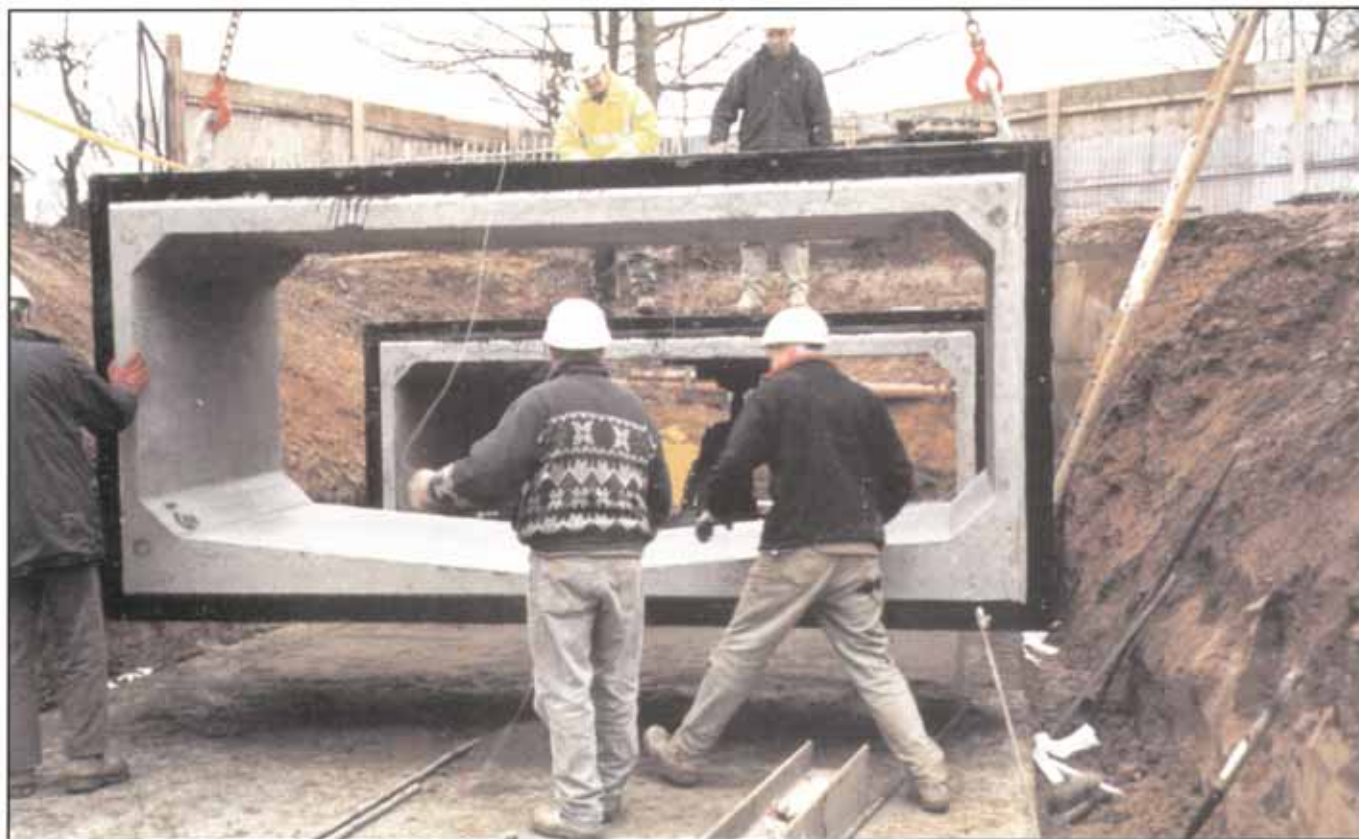
Below: A Brierkrete precast culvert section is maneuvered into position.
