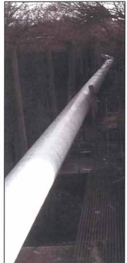
Denso Steelcoat 700 System protects the exposed Transco pipeline.
