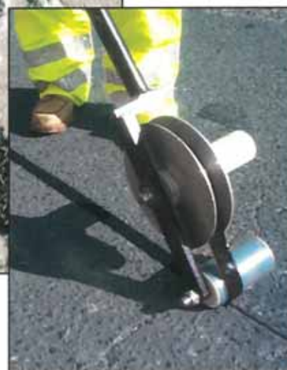
Simple, fast application of the new Denso Skid Resistant Overbanding Tape by special applicator machine.
