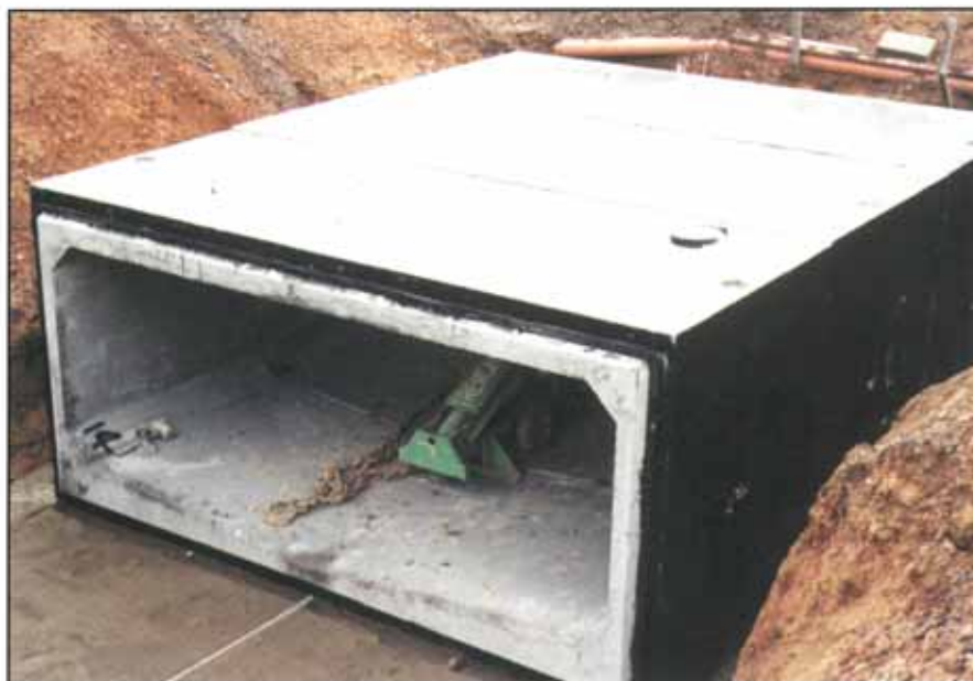
Above: The Tokstrip jointed attenuation tank starts to take shape.
