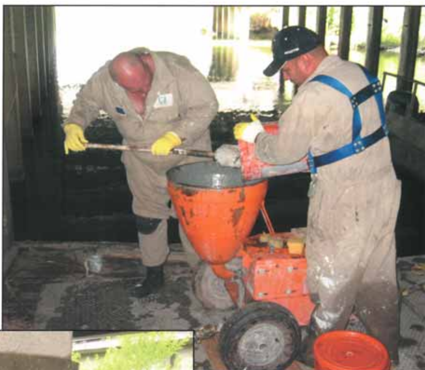
Above: Mixing the SeaShield 500 Epoxy Grout.
