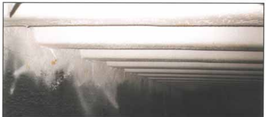
The protected bridge steelwork showing the confined access conditions.
