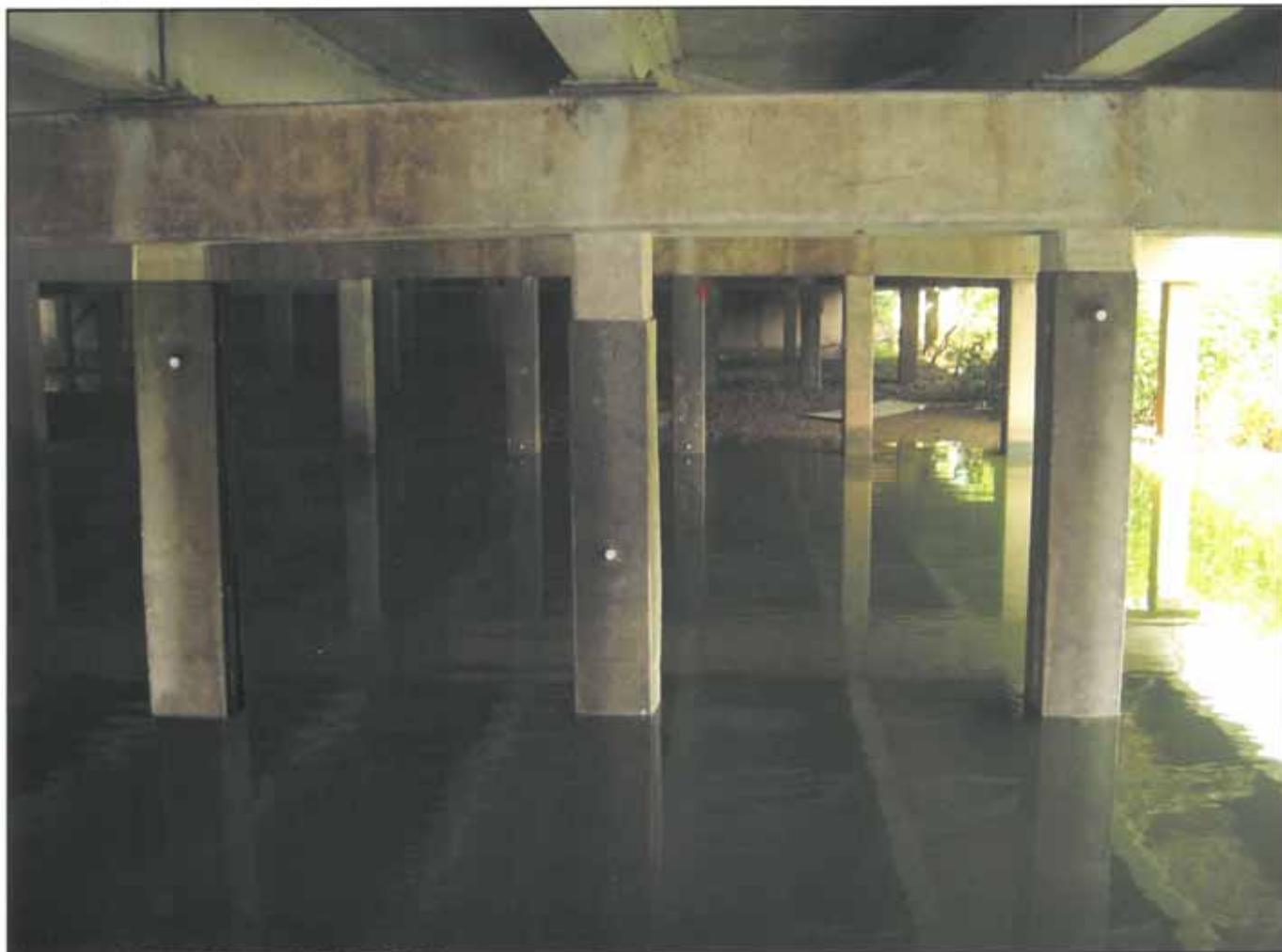
View under bridge of SeaShield 500 protected piles
