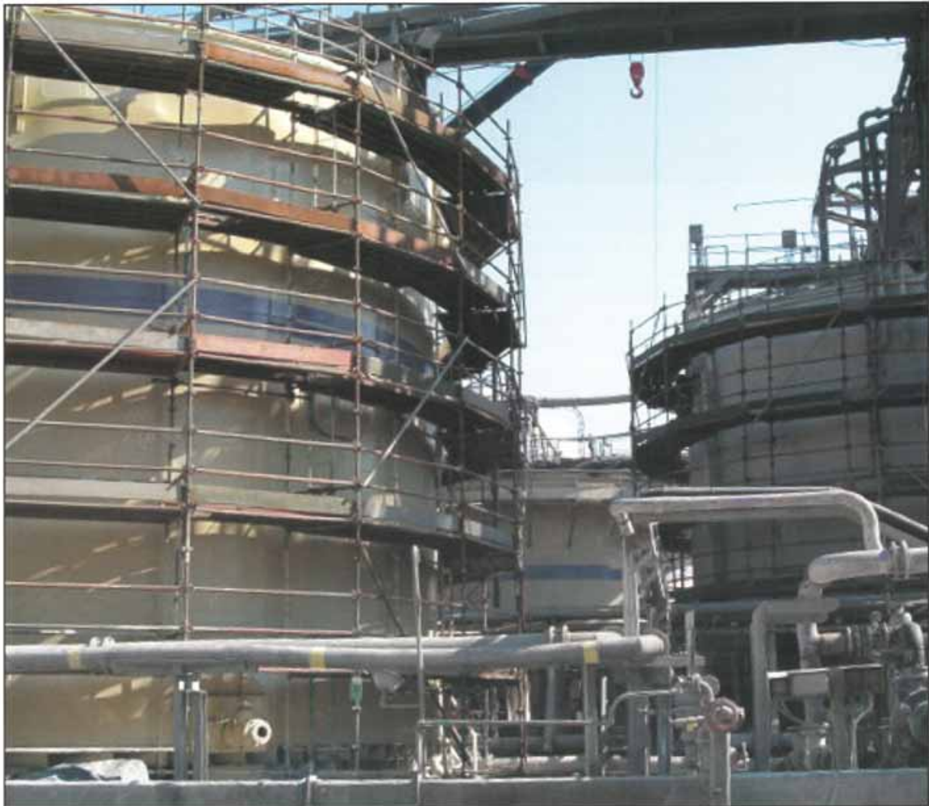
Two of the tanks during application of the Denso Steelcoat 700 System.
