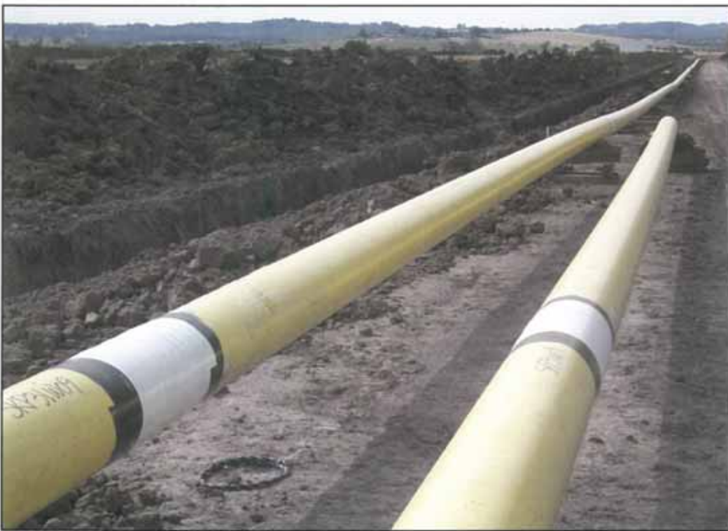
Denso 3 Ply Butyl Tape System protect pipe joints on the Bassgas Onshore Project.
