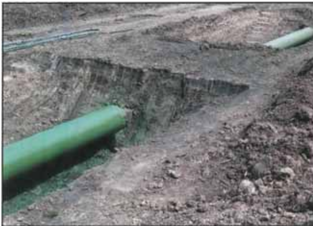
Spray applied Protal 7200 protects 600 linear feet of 36" diameter pipe.
