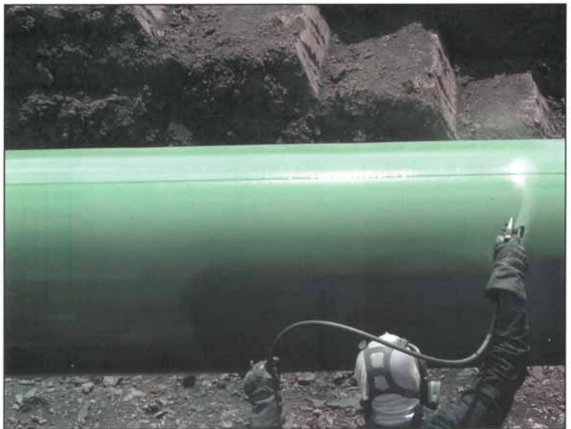
Spray applied Protal 7200 protects 600 linear feet of 36" diameter pipe.
